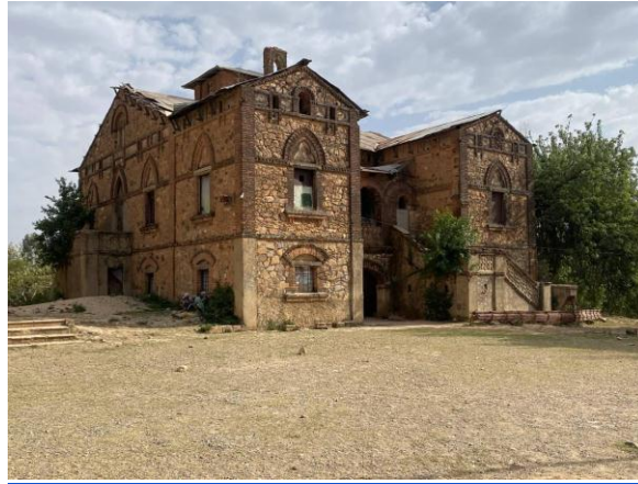
Figure 20. picture showing Italian consulate building (2024)
