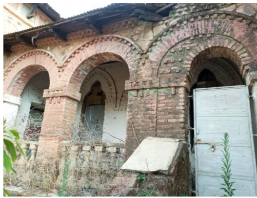
Figure 24. image showing arches in the balcony
