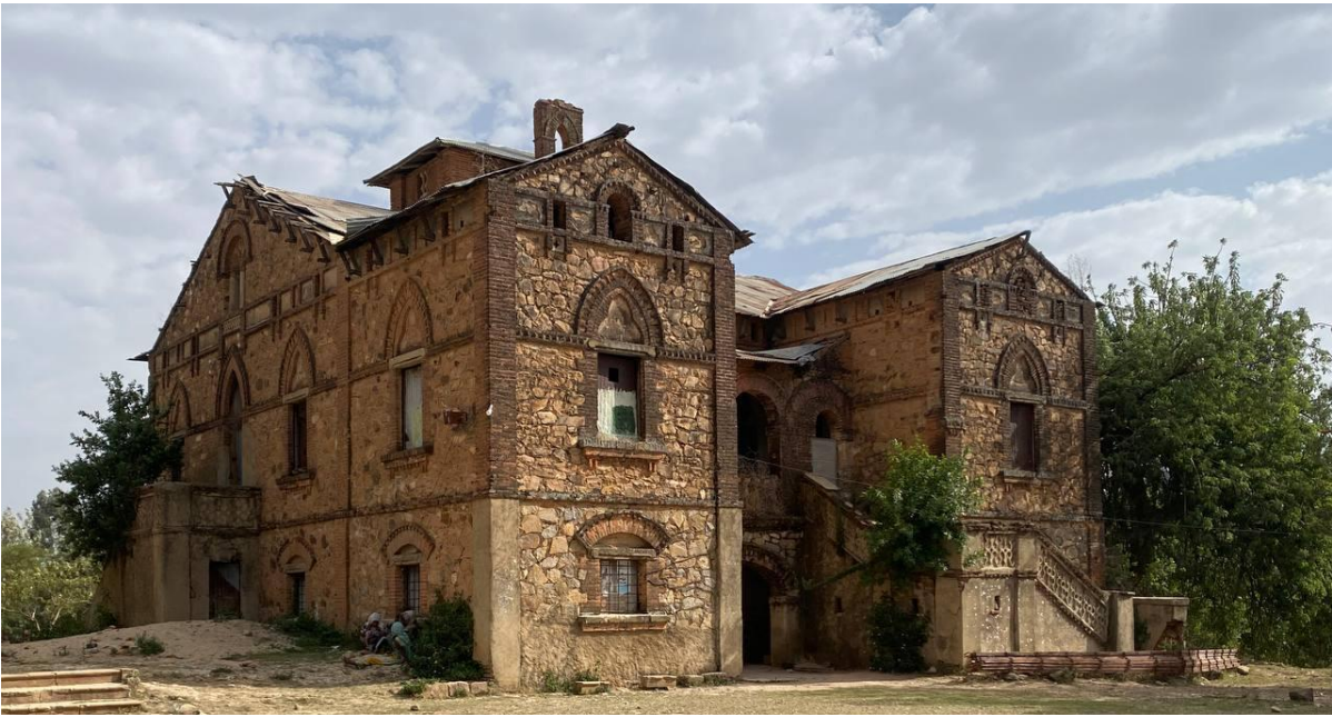
Figure 44. image showing missing windows
