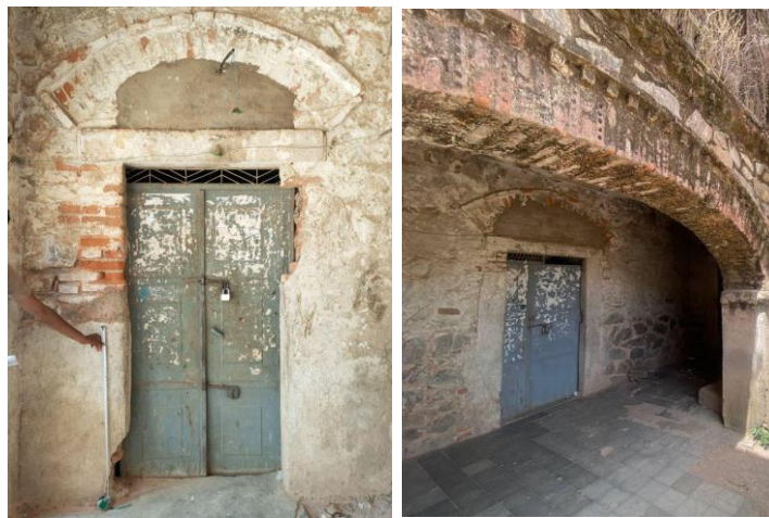
Figure 43. images showing replaced doors
