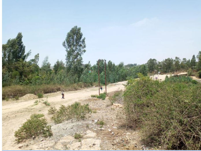
Figure 17. Image showing the new road under construction
