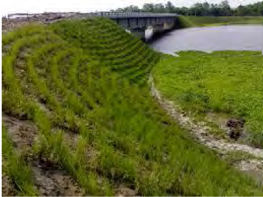
Photo 7.2 Vetiver grass for erosion protection (Source; internet )
