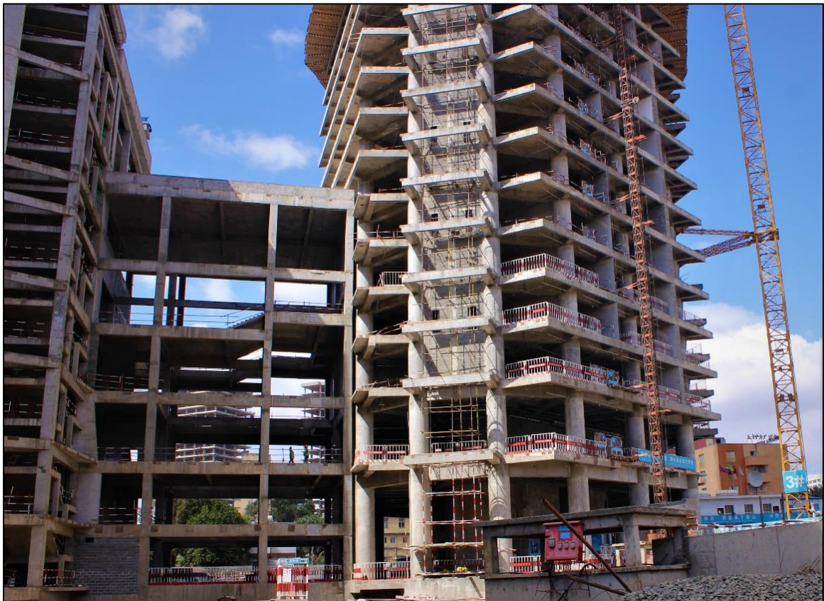
Figure 20: CBE-HQP Main Tower, Pedestrian Bridge, Elevator and Tower Crane Visible
