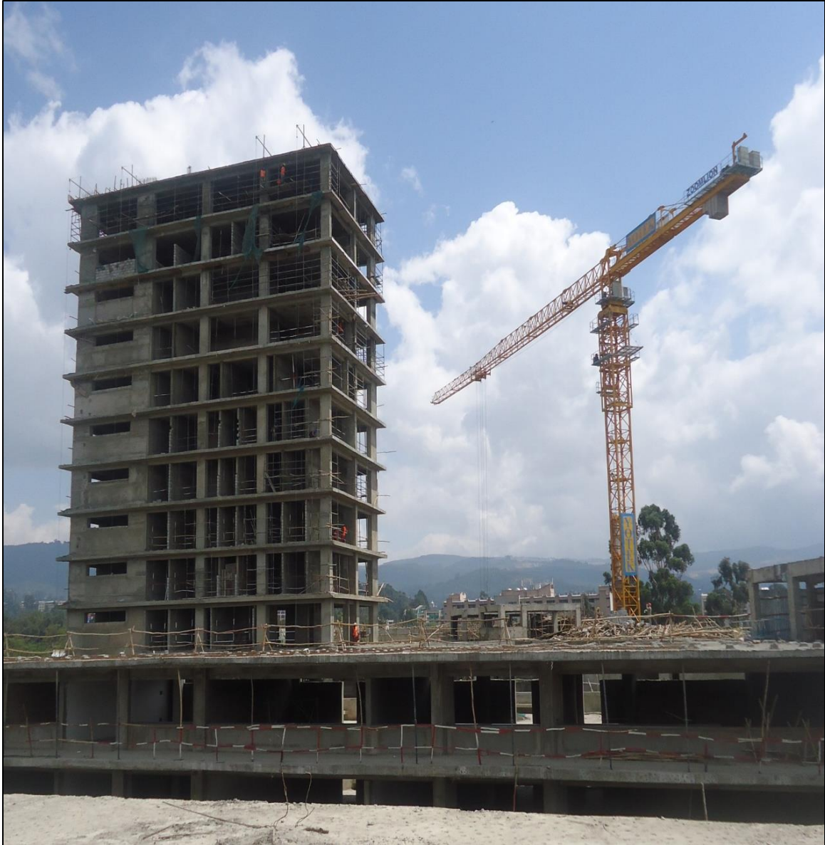
Figure 1: AAU Forum Building Crane (Courtesy of Yotek Construction)
