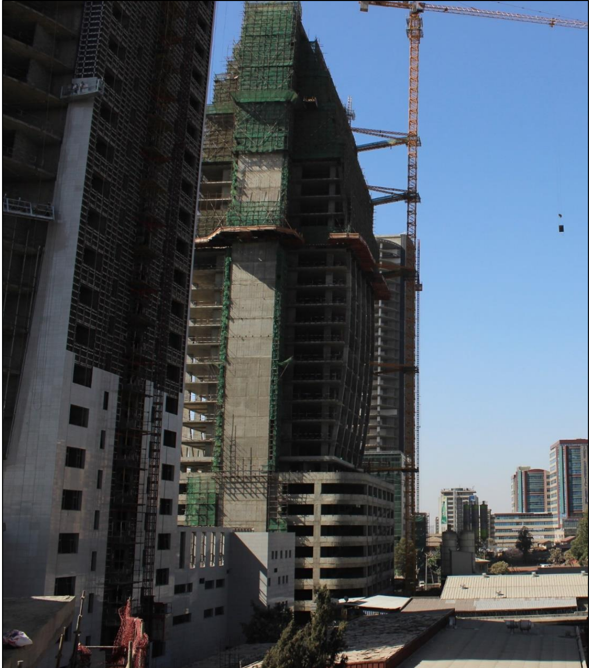
Figure 33: Side Profile of ZB-HQP Building
