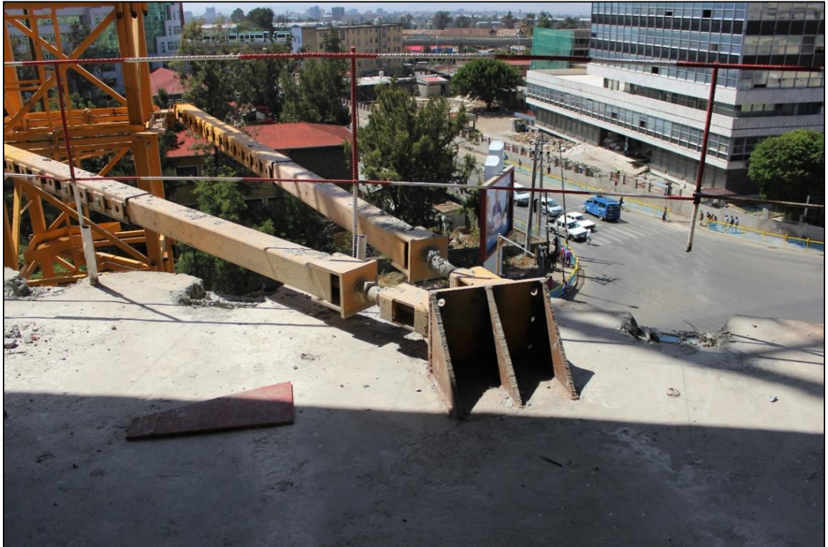
Figure 45: UB-HQP Crane Anchoring to Slab
