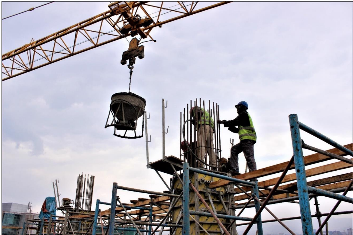
Figure 27: NI-HQP Concrete Transportation with Crane and Bucket
