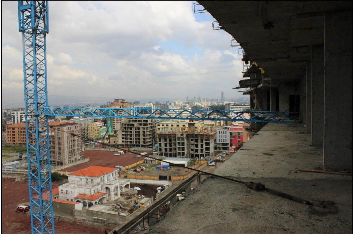
Figure 63: Anchoring of Marriott Hotel Tower Crane Using Wires
