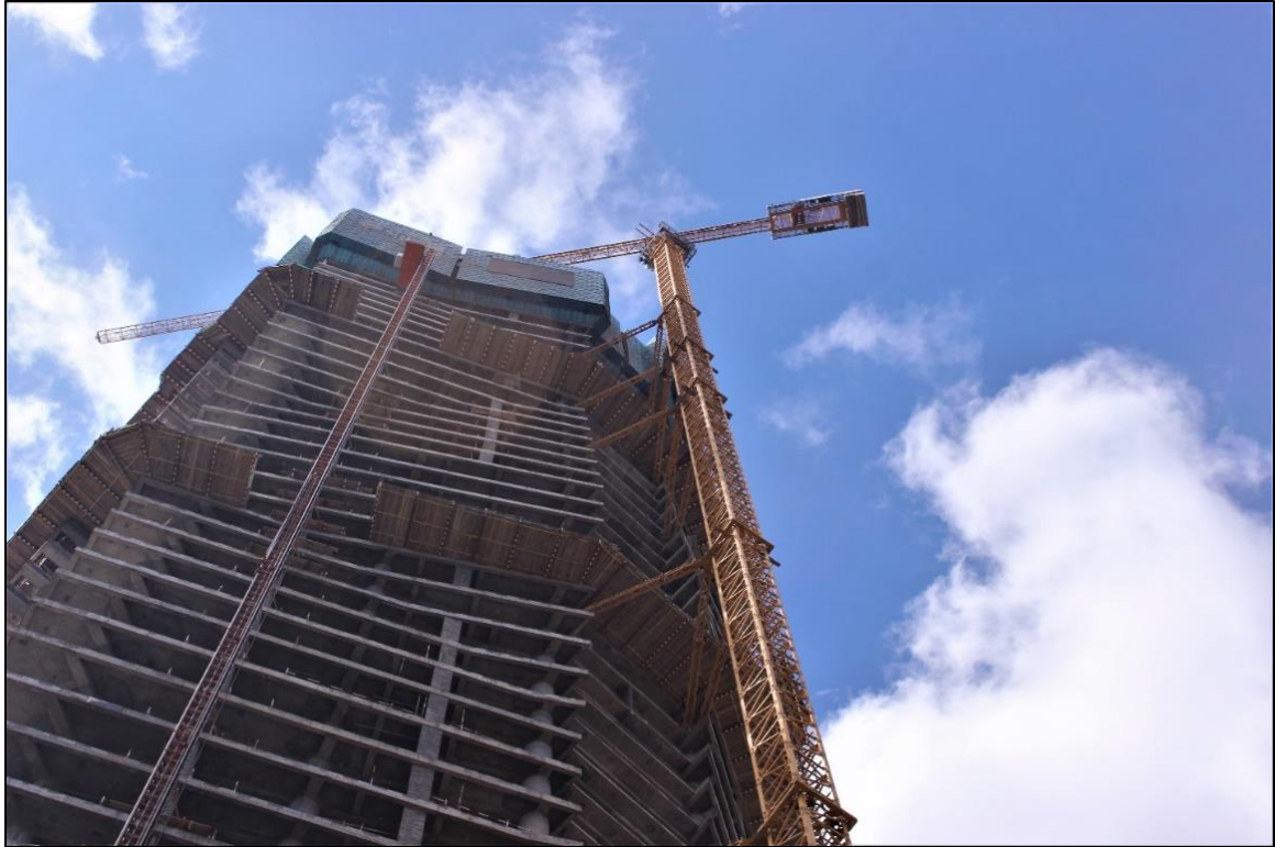
Figure 19: CBE-HQP Main Tower, Crane and Construction Elevator Visible
