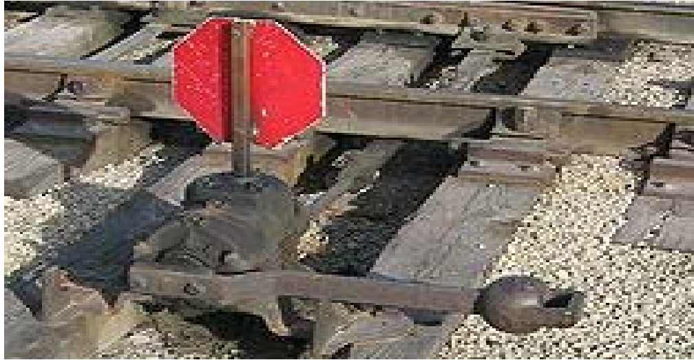
Figure 2.6: low switch stand.
