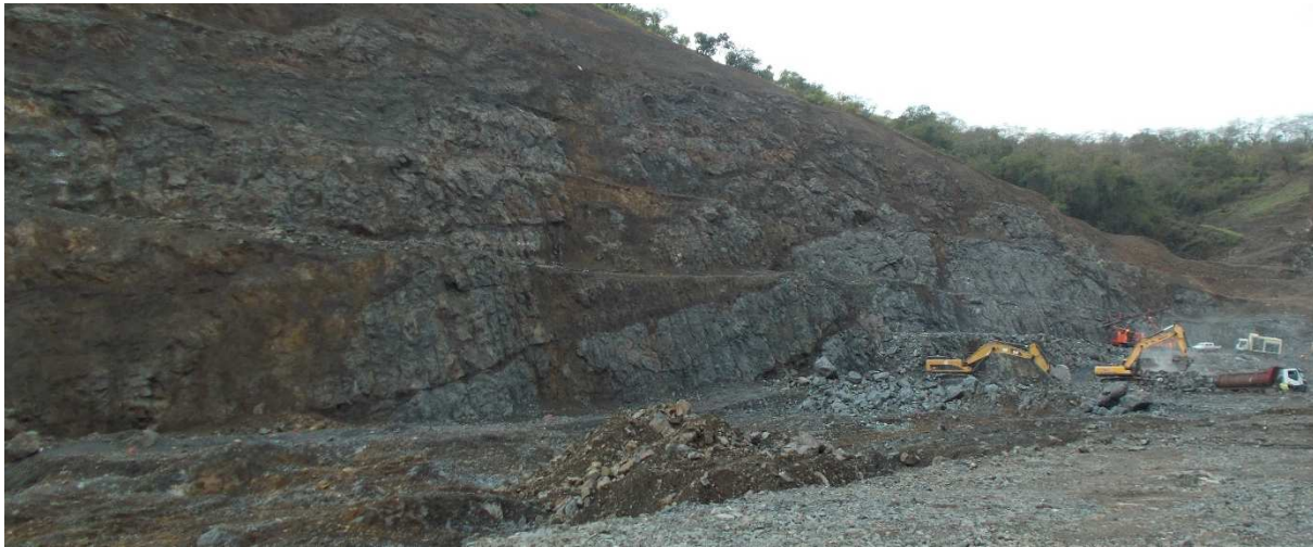
Figure 7.21. J2 joint with thick infilling on the abutment slope
