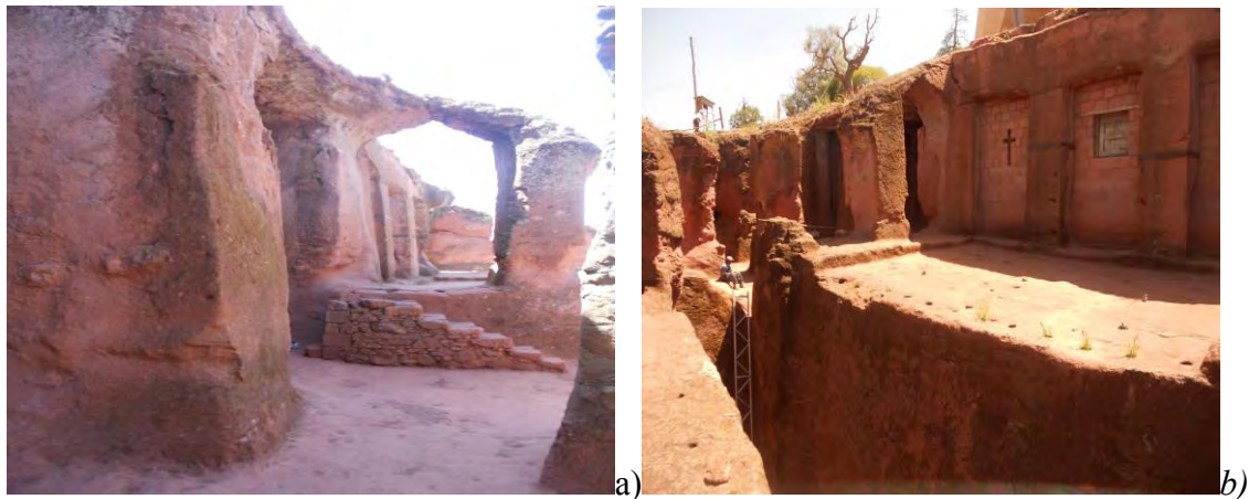
Figure 23: Bete Merqorios Church a) from N-W Direction b) from S-W Direction
