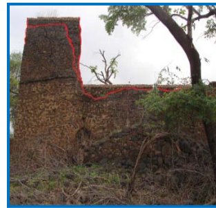
Figure 44: Masonry works-re-pointing and capping (Photo by Feyissa H, 2016).
