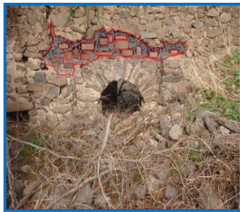
Figure 44: Masonry works-re-pointing and capping (Photo by Feyissa H, 2016).
