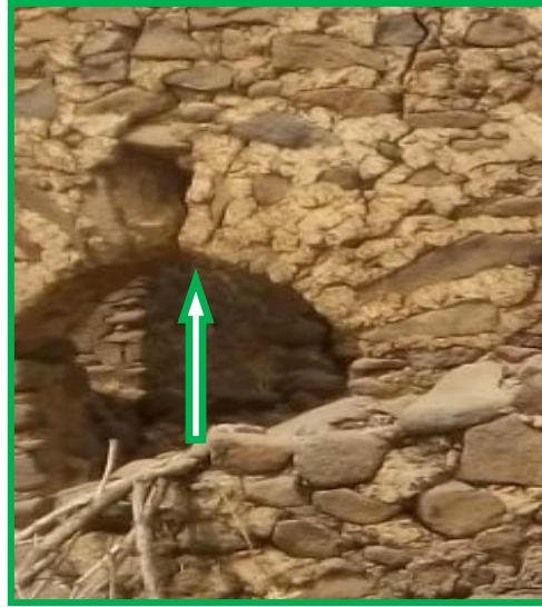
Figure 36: Sunlight cracking view on enclosure (a) and lost stones on joint part of the castle (b) (Photo by Feyissa H, 2016).
