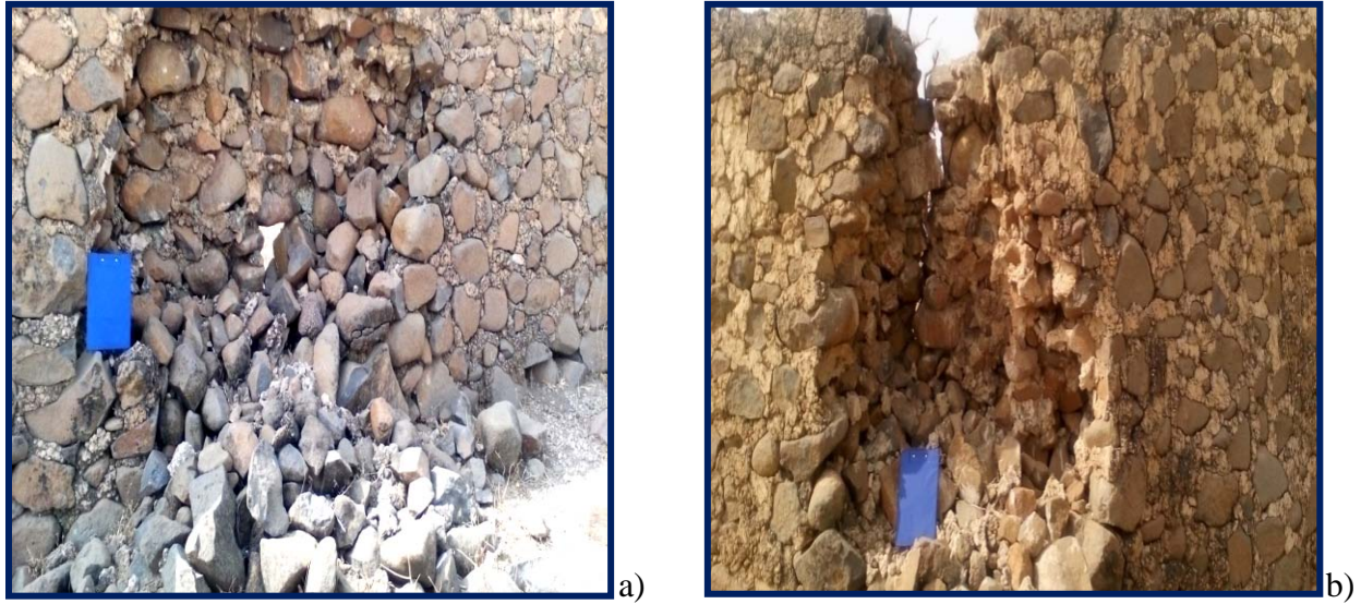
Figure 35: Small destruction before a year (a) and after a year (b) (Photo by Feyissa H, 2016).
