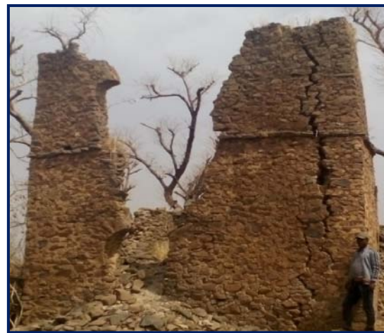
Figure 37: Comparison showing destroyed western wall-direct sunlight exposed (a) versus better saved of northern wall (b) (Photo by Feyissa H, 2016).
