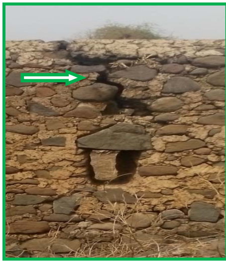
Figure 36: Sunlight cracking view on enclosure (a) and lost stones on joint part of the castle (b) (Photo by Feyissa H, 2016).
