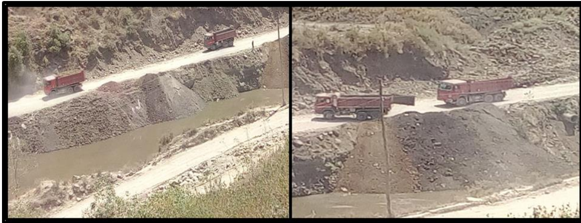
Figure 5.4. Trucks disposing cleared upper soil from quarry in to Akaki River.
