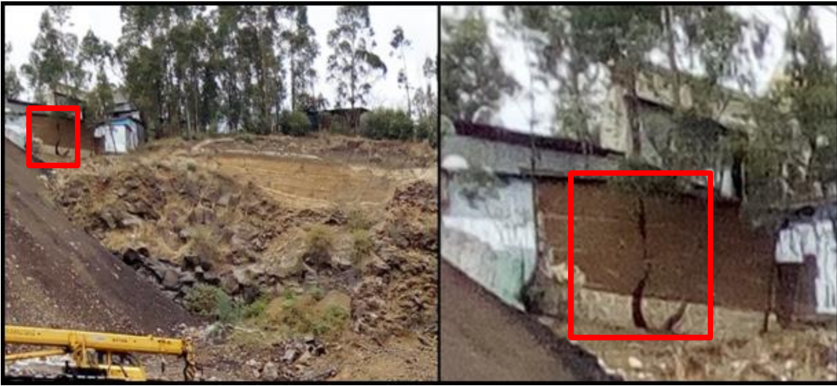
Figure 5.19. Cracked house due to quarry blasting.
