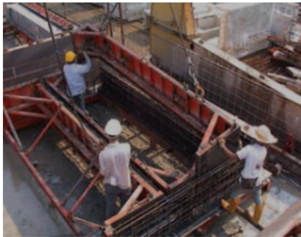
a) Assemble the mold components
