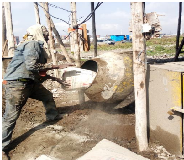
a) Batching of cement on transit mixer
