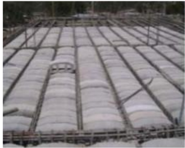
b) Ribbed beam installation with blocks
