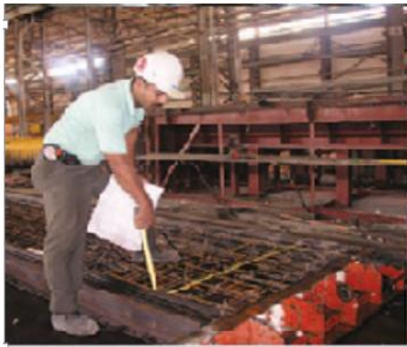
a) Check rebar spacing and lap length
