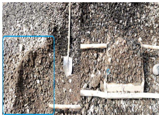
b) Batching and grading of coarse aggregate
