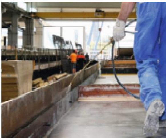
a) Application of mold releasing agent
