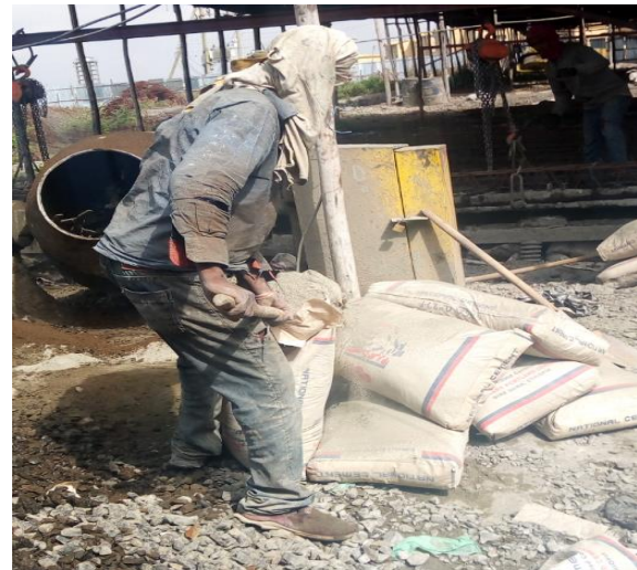
b) Applied extra cement on the same mix
