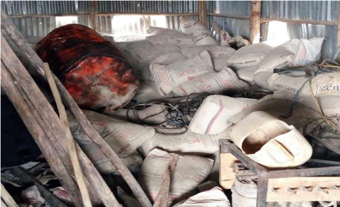
Figure 4.8 Cement storage practice on the ribbed beam manufacturing shade through MSEs (picture taken by the researcher).
