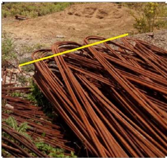
a) Inaccurate rebars cutting practice
