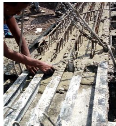
c) Vibrate the casted concrete
