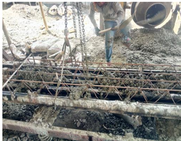
b) Random placing of concrete on the mold
