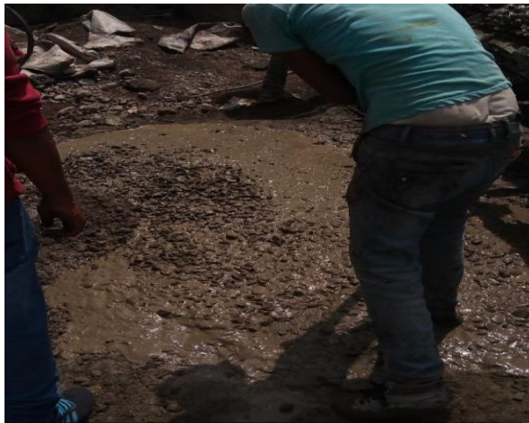
a) Putting of concrete on the unsafe ground
