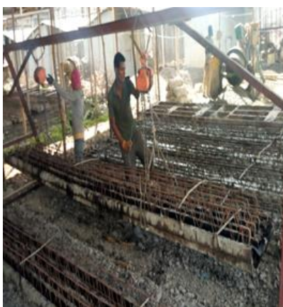
a) Lifting and moving of the entire mold component
