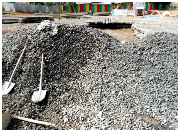
b) Storage practice of coarse aggregate
