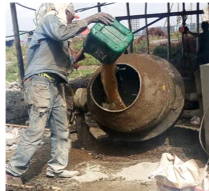
c) Application of mixing water
