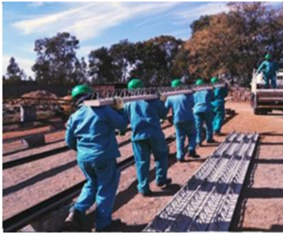
a) Precast ribbed beam handling
