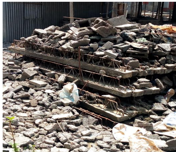
b) Beams stored with wasted materials.
