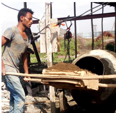
a) Over batching of sand
