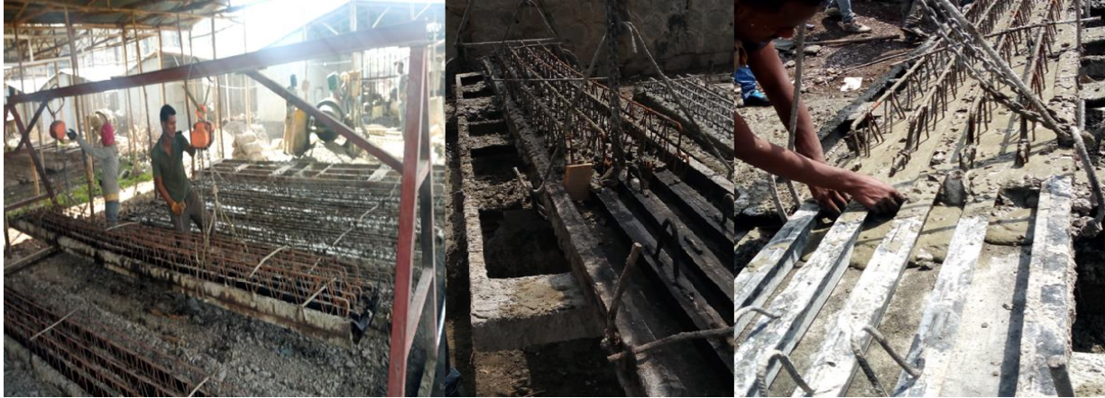
Appendix 4.3: Views of molding, fixing rebar and casting fitting practice
