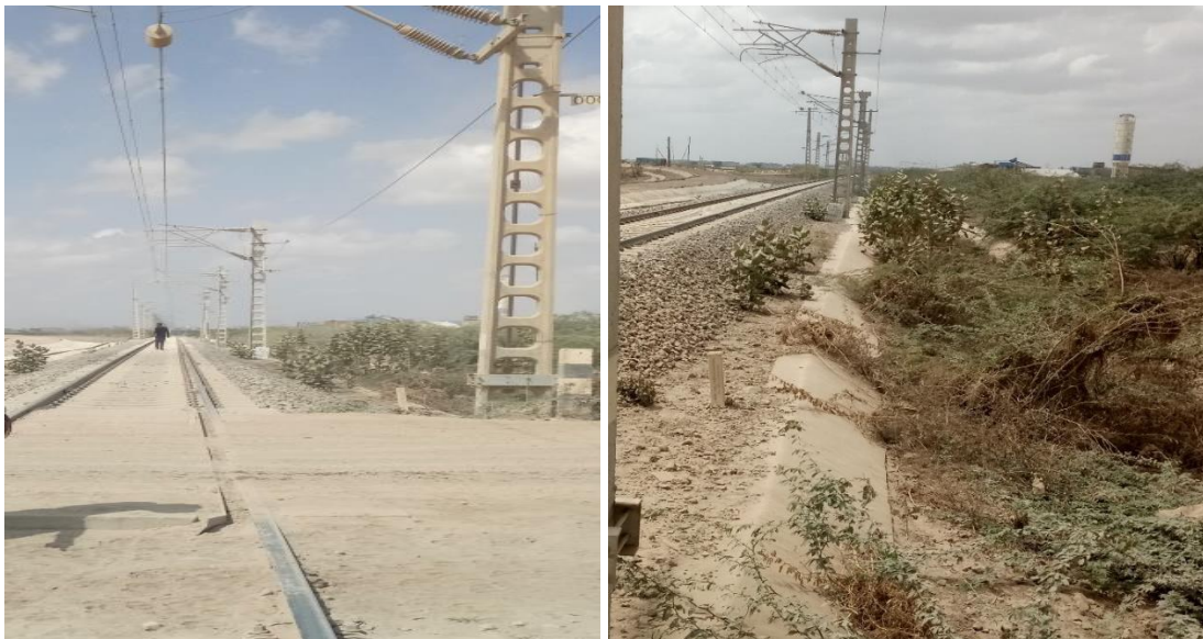
Figure 3.2 Fouling Ballast on the Left and Sand Contamination Spots on the Right Side
