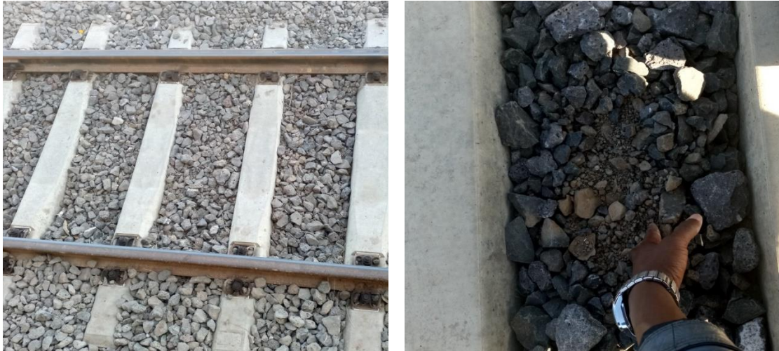
Figure 3.2 Fouling Ballast on the Left and Sand Contamination Spots on the Right Side
