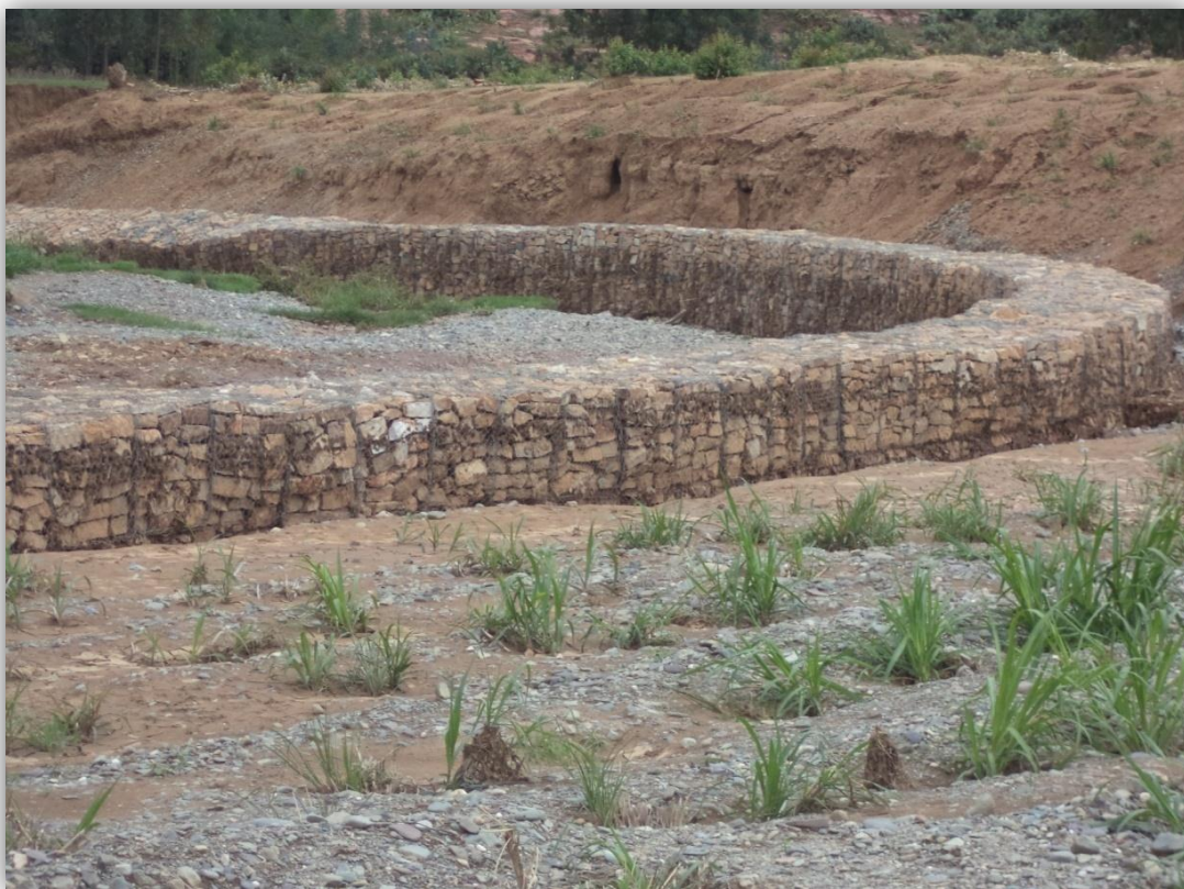
Figure 23. (a) and (b) Example of conservation mechanism in Hayk Mesahil stone bunds
