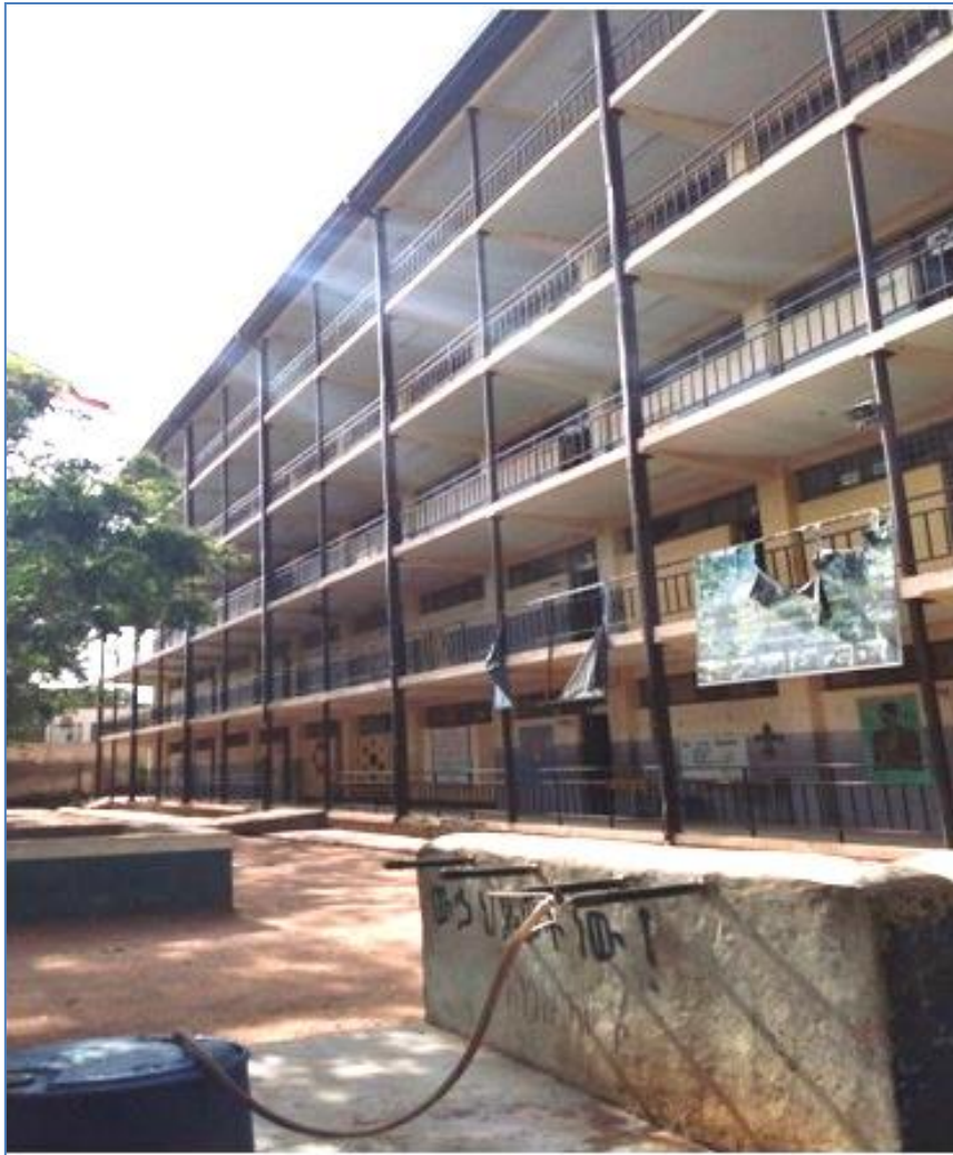
Figure 3.1 Existing building over view
