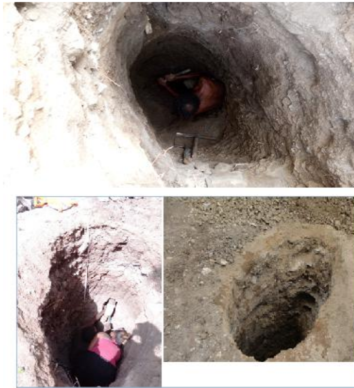
Figure 4.2 Pit 1 and 4 excavations around the building and taking soil samples
