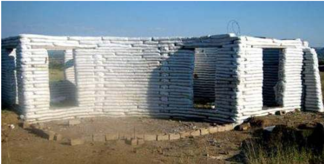
Fig.3.7 House made of earthen bags [20]
