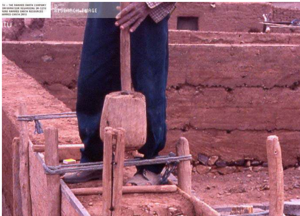
Fig. 3.6 Compacting of mud in the wall-mould rammed earth [9]
