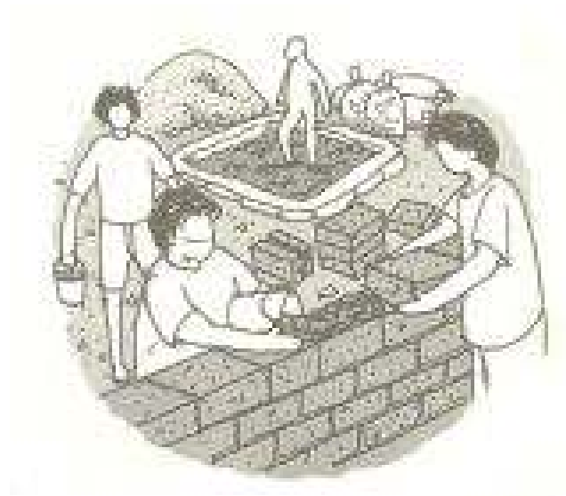
Fig.3.2 Bonding sun-dried adobe brick with clay mortar [16]
