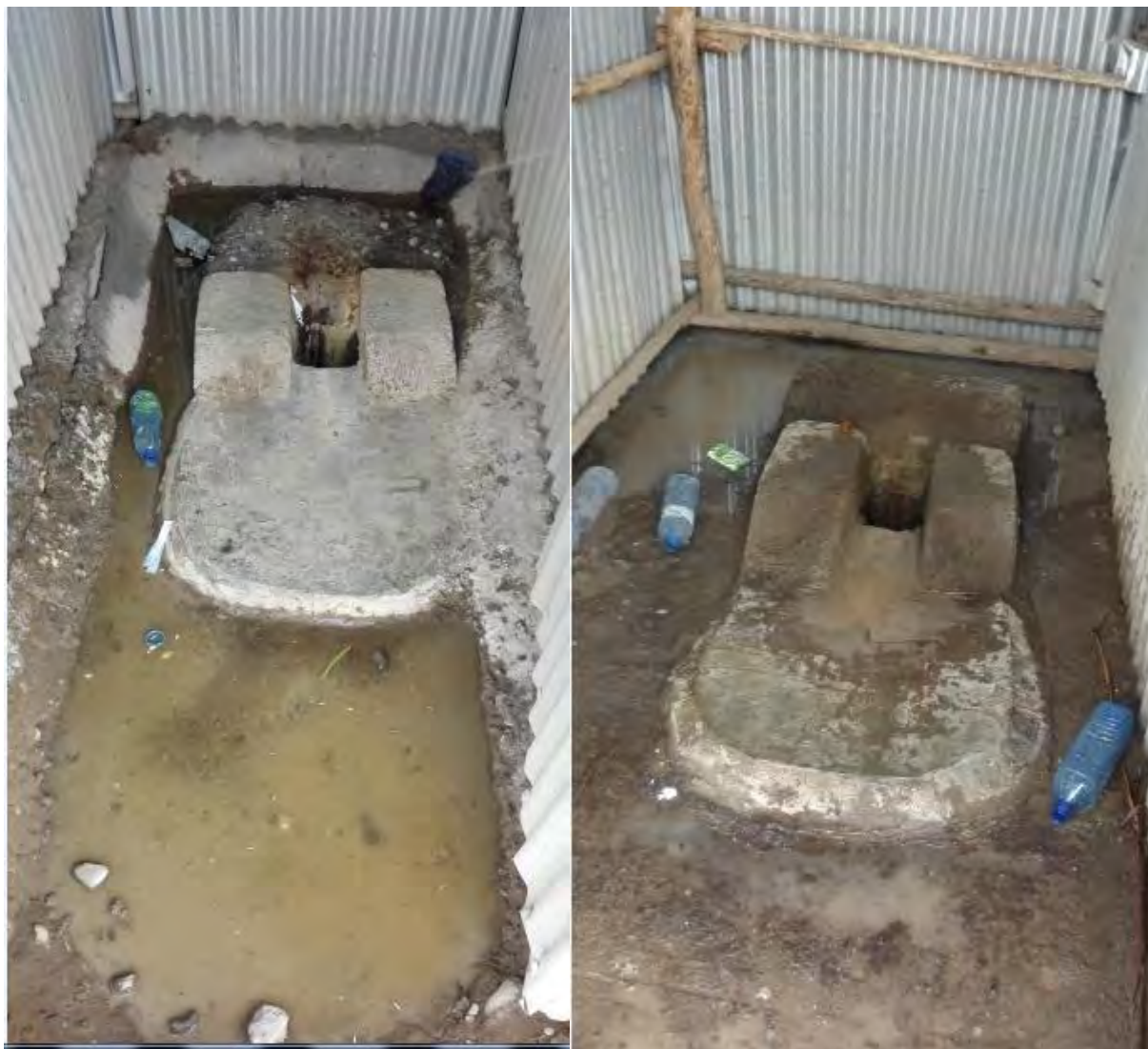
Figure 32: A sample photo of latrine used by the trainee with full of dirty overflowing sewage and without slap.
