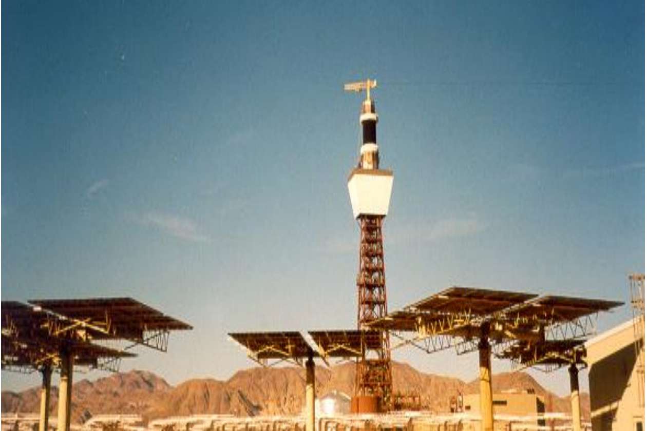
Figure 1-1: Solar Two Central Receiver Power Plant
