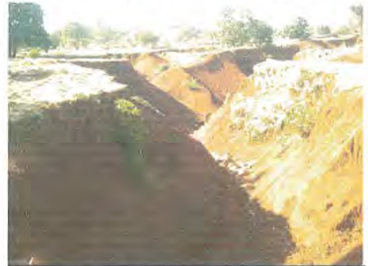
Figure 10: Gully erosion in Dendegeb
