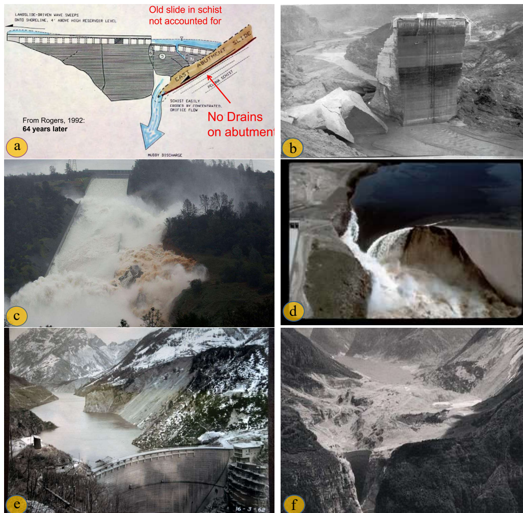
Figure 3.1: Dam failure cases due to geological problems: (a) and (b) St. Francis dam failure, 1928, (c) spillway failure of Oroville dam, 2017, (d) Teton dam failure, 1976, (e) and (f) Vajont dam, 1963.
