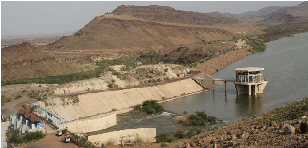
Figure 6.44: Tendaho earthfill dam(left), spillway (right) and intake tower in the middle.
