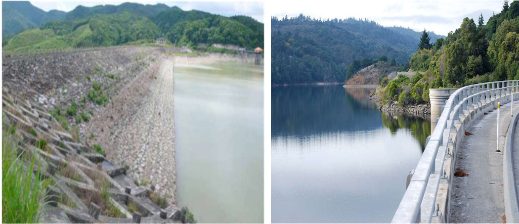
Figure 2.1 : Upstream view of Aratozawa rockfill dam in Japan (left) (Hinks et al., 2012) and Lower Crystal Springs gravity dam that survived the 1906 M 8.3 San Francisco earthquake and M 7.1 Loma Prieta earthquake of 1989) (right) (USCOLD, 1992).
