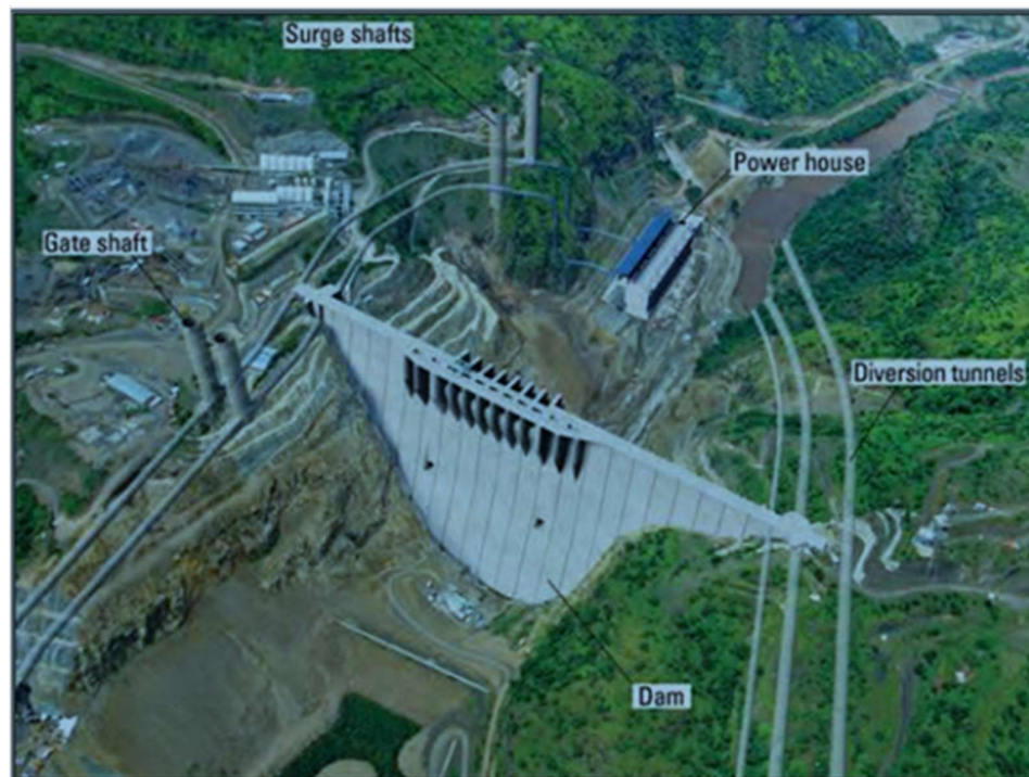
Figure 6.3: Gibe III project site model showing dam and appurtenant structures (EEPCCO, 2009)
