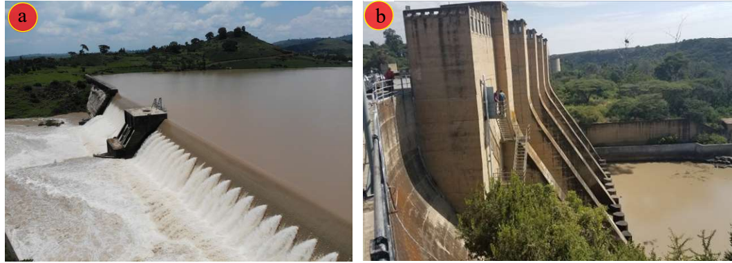
Figure 5.4: The oldest hydropower dams grouped under high seismic risk class: (a) Aba Samuel dam, (b) Koka dam
