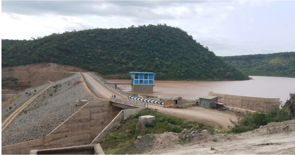
Figure 6.32: Gidabo dam with spillway at left abutment and irrigation intake tower.
