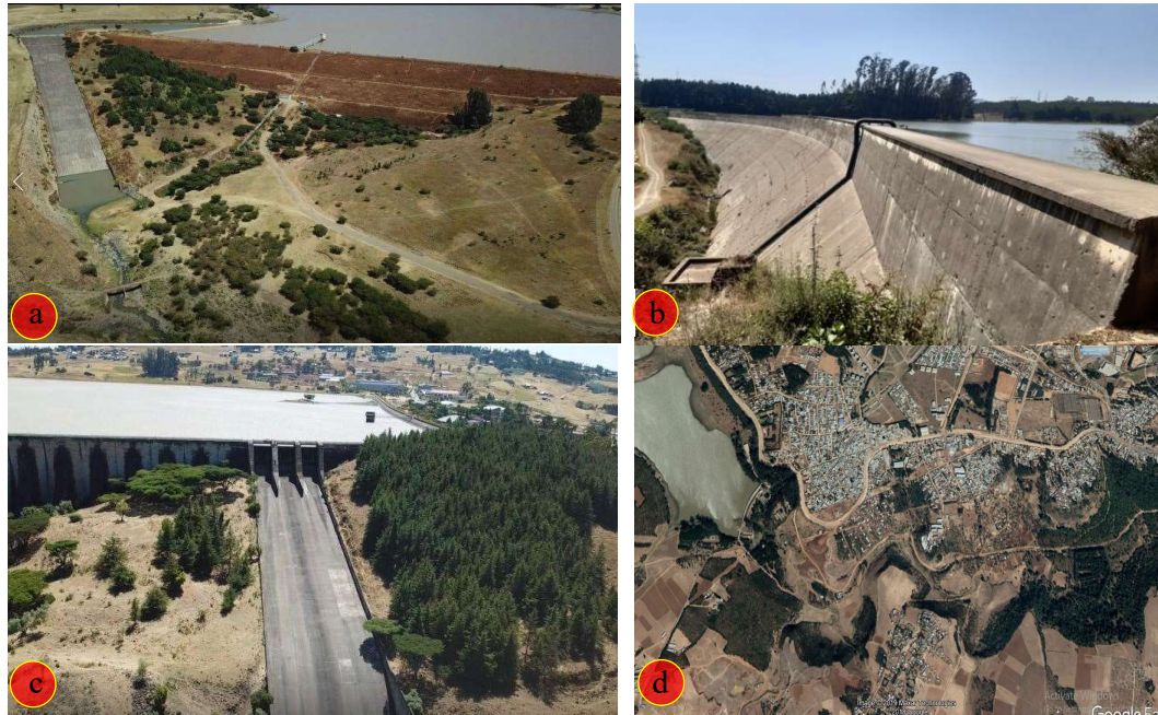
Figure 5.3: Addis Ababa City Administration dams and downstream flood risk zone: (a) Dire dam, (b) Gefersa gravity dam, (c) Legadadi dam, and (d) part of Burayu town in the flood zone of Geferesa dam
