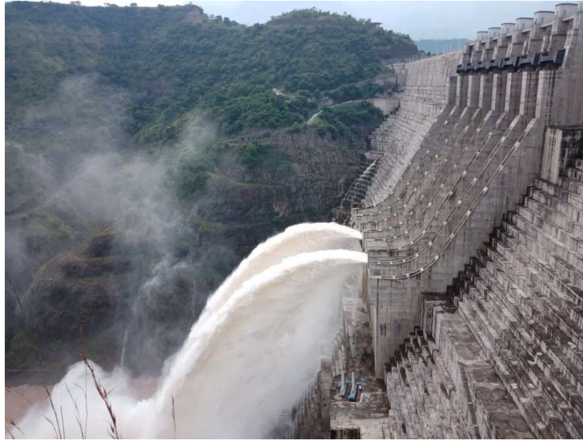
Figure 6.9: View of Gibe III dam showing overflow and non-overflow dam sections: the two MLO are spilling
