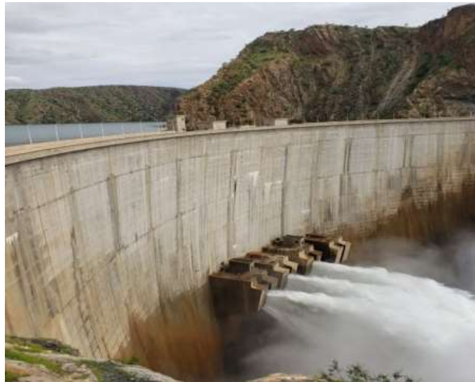
Figure 6.54: View of downstream face of Tekeze arch dam with four orifice spillways
