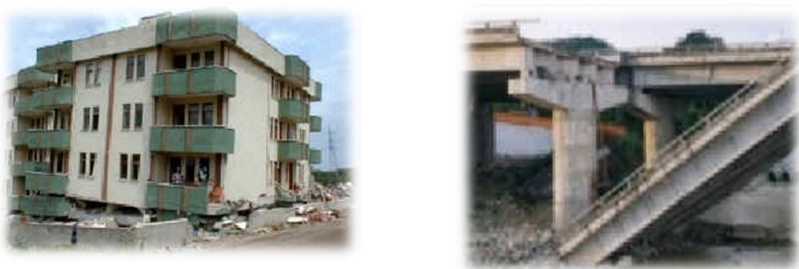
Figure 2.5 The 1961 earthquake destruction: structures collapsed in Addis Ababa city.
