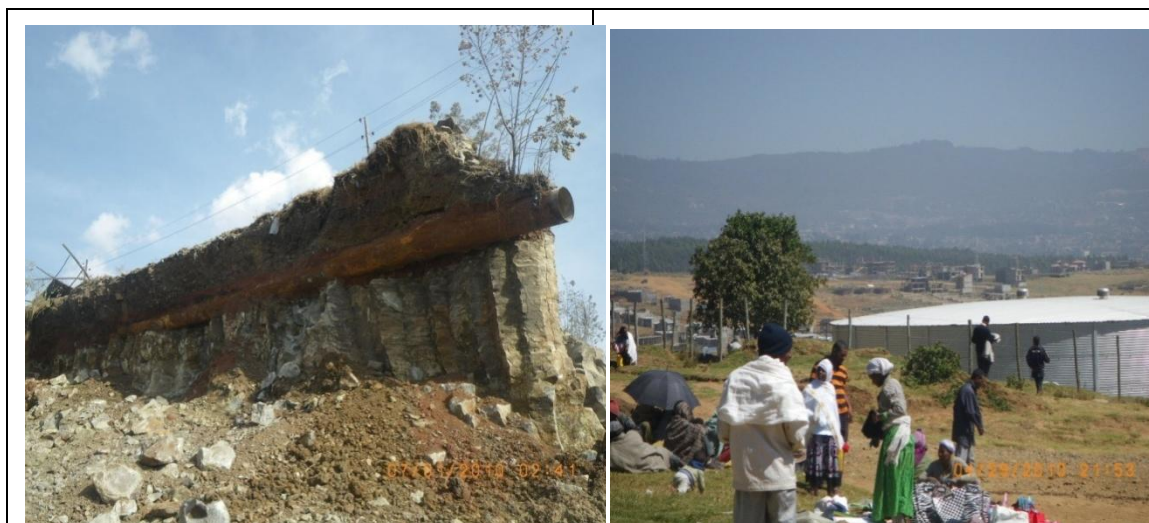
Plate 4.5 Human made infrastructures/ utilities (abandoned water mains and gravity water tankers, with a capacity of 1.5million m 3 ) constructed on hilly areas; potential to develop subsurface pore water pressure due to seepages; considered as triggering factor for land instability; Yeka and Nefas Silk Lafto sub cities, A.A.
