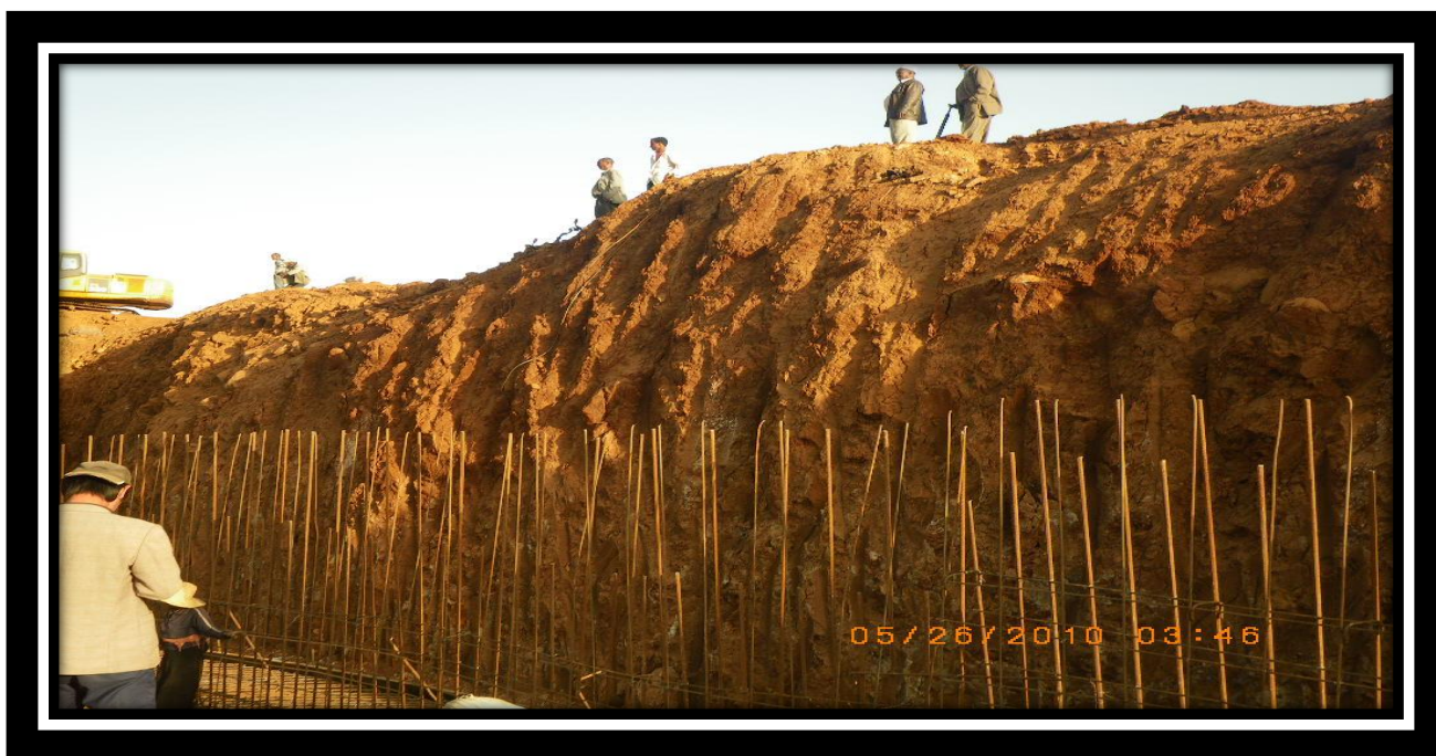
Plate 1.5. Residual soils: weathered brown to red silt clay soils(Eutric Nitisols) found in Gulele as thick as 12m; sections exposed during ring road construction (Gojam Ber, Gulele sub-city, AA), 2010
