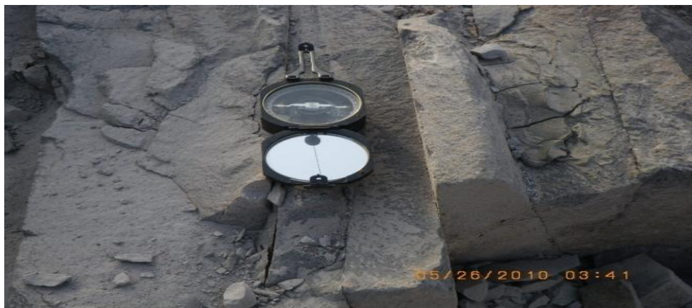
Plate 4.2 Major discontinuities seen on fissured fresh intrusive dome like basalt exposed in Gulele ring road construction project, and has been oriented similar to the main axis, i.e. N-E trending pattern, Gojam Ber area, Gulele sub city, A.A. See the compass needle directed towards N_S axis.
