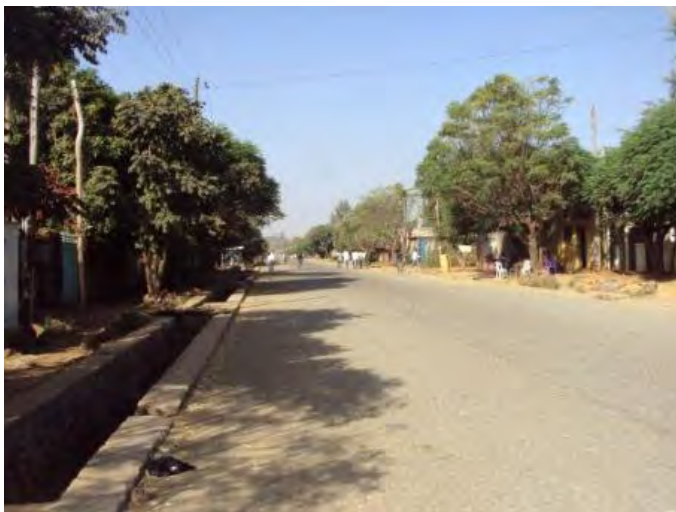
FIGURE 4: Sub arterial road inside the neighborhood
