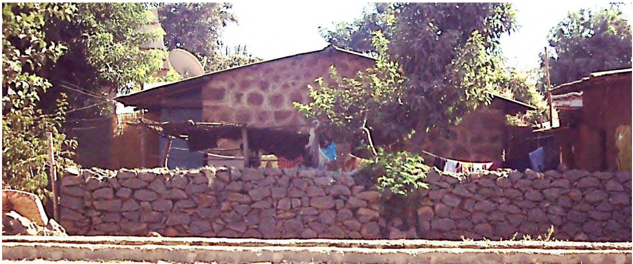
FIGURE 8: Main core house
