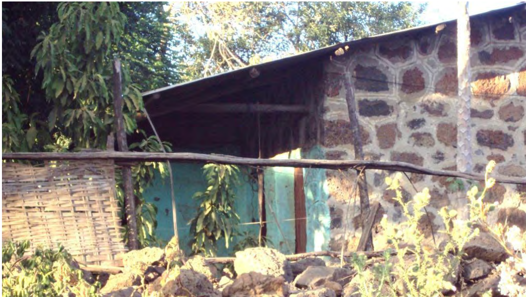
FIGURE 11: Maintenance in the main core house
