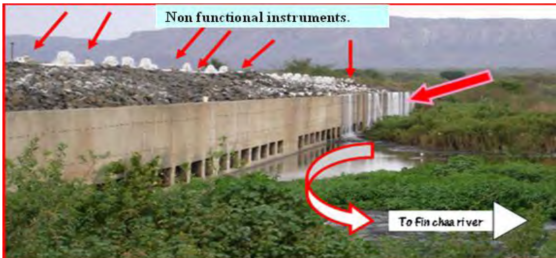
Figure 6. Industrial waste water treatment plants near the factory. (Source Ahimed Amdihun 2005)
