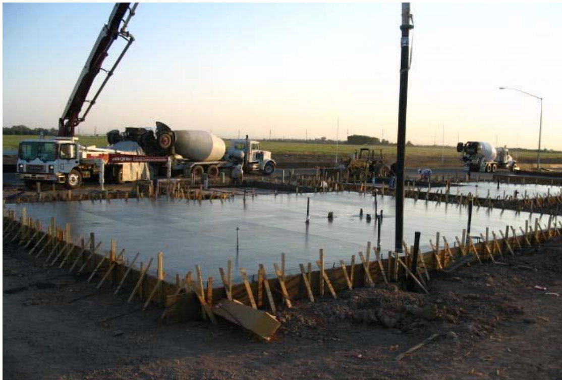
Photo 2.4 after pouring concrete
