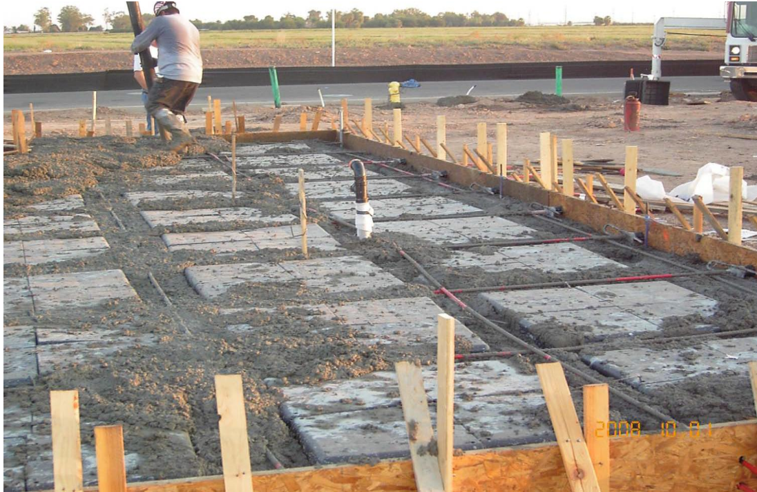
Photo 3.3 Pouring the concrete
