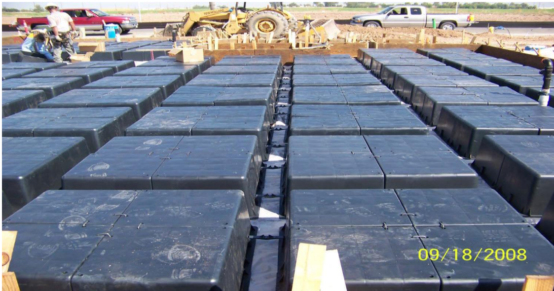
Photo 2.1 Lay out waffle boxes and connects with plastic clips
