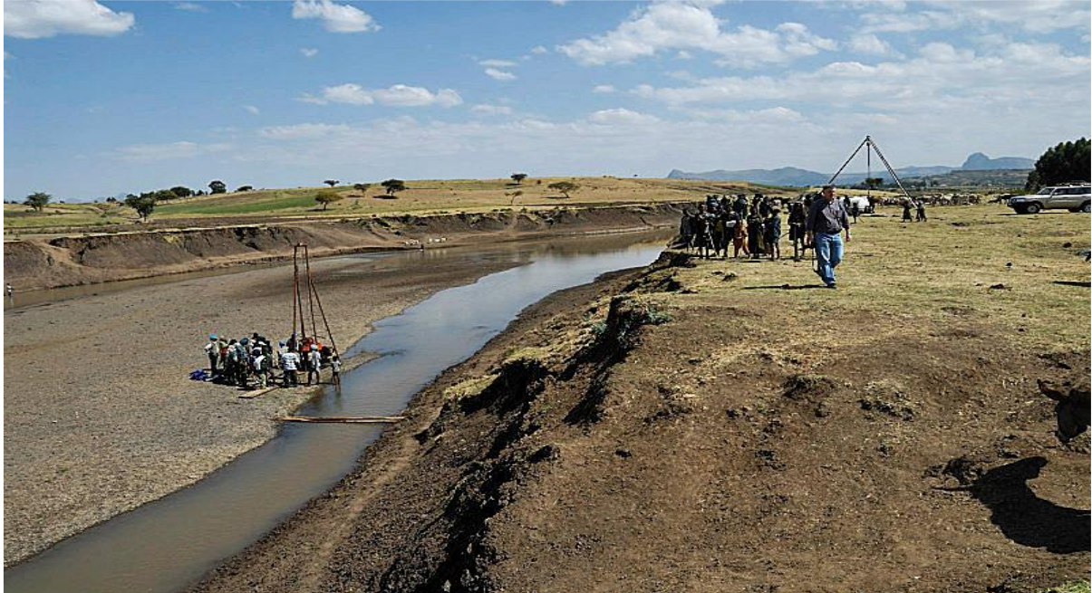
Figure 3.0.6 Geotechnical investigation of the weir site (Source: TAHAL consulting engineers Geotechnical Report annex B.3.2.1)
