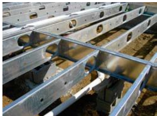
Figure 2-2 Floor joist
