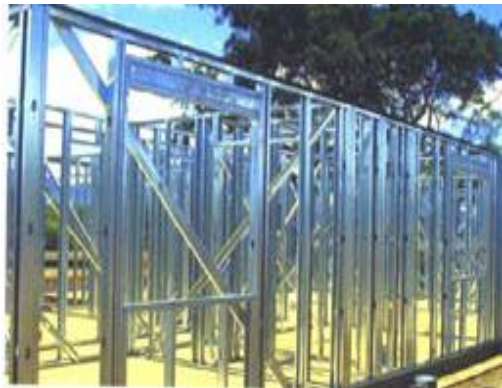
Figure 2-1 Wall framing
