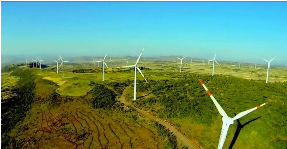
Figure 3-5 Adama wind project site
