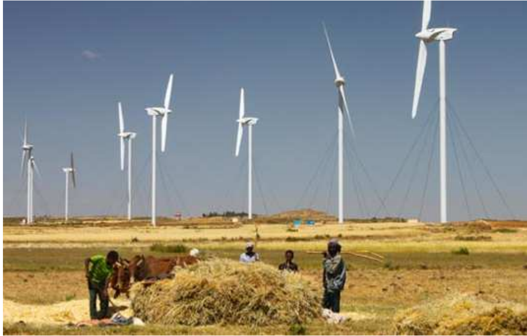
Figure 3-4 Ashegoda wind project site
