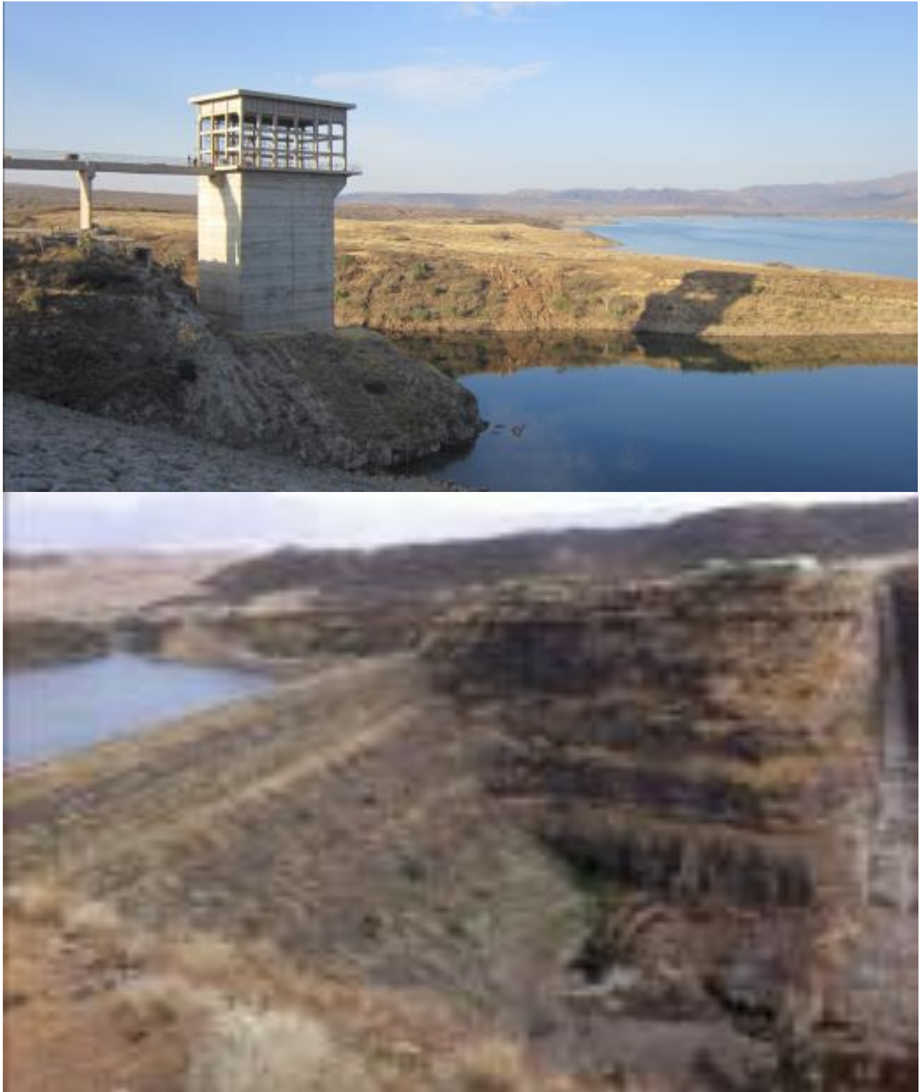
Figure 3.3 Kesem River and its dam (GKM Consultant project summary)
