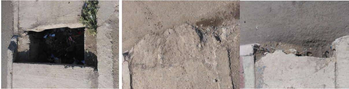
Figure 5.3 Condition of Manholes inlets
