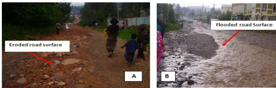
Figure 2.5 highly eroded road (A) and flooded road surface (B). Source (Danachew A, study of urban drainage system in Addis Ababa, Yeka sub-city.2011..)
