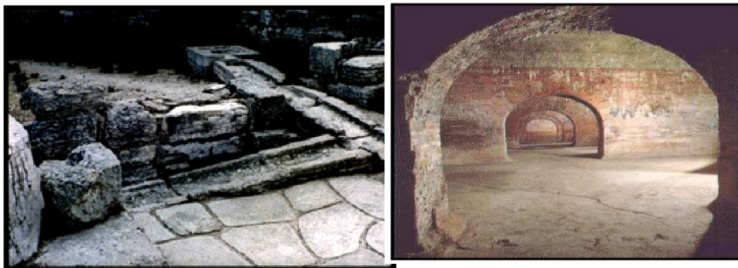
Figure 2.1 Minoan storm drain at Knossos dating to 1500 BC. (Daedalus 2002) at the left and picture of Roman cistern in Fermo, Italy.
