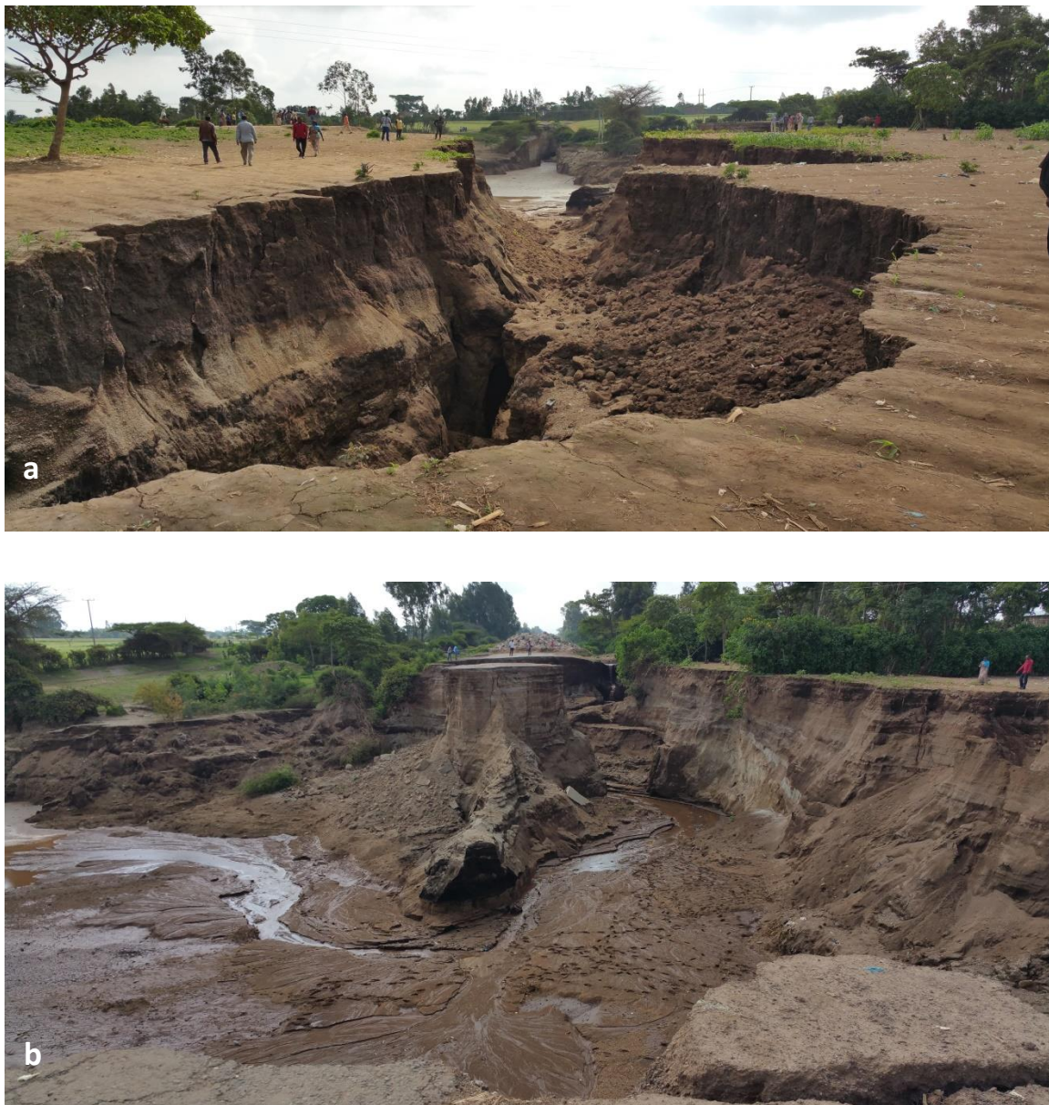
Figure 1.1. (a).The Ground fissures that developed at Oine Chafo Umbure on the Shashamane-Aje road in the summer of 2016 and in (b) is old asphalt road in the foreground.
