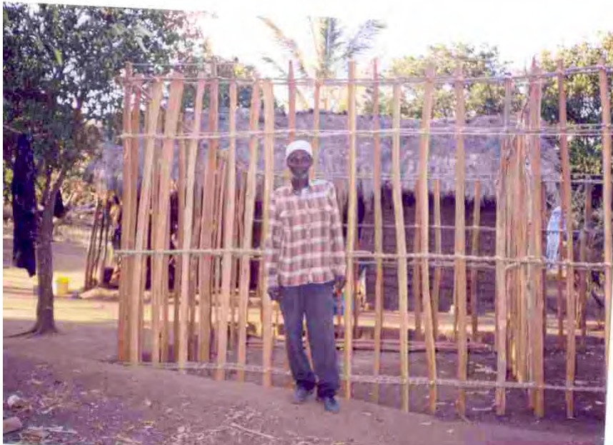
Plate 5: A house under-construction using Brachylaena huillensis poles in Fulwe village.
