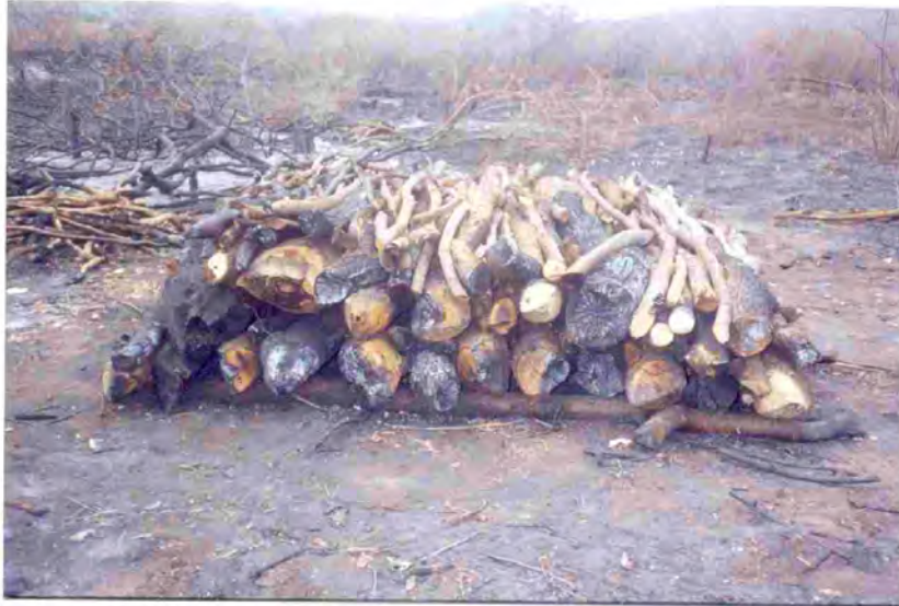
Plate 3: A charcoal kiln under construction in the forest reserve
