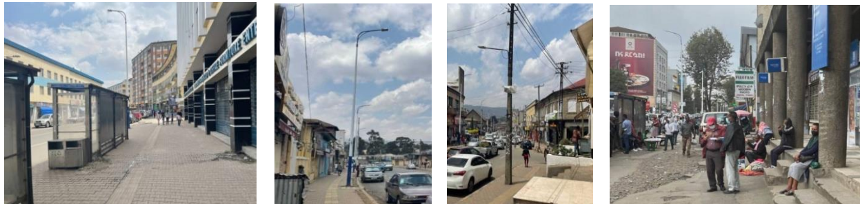
Figure 52: Presence of Street Furniture along Halieselassie Street sidewalk
