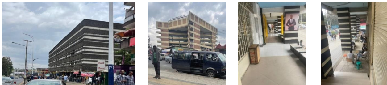
Figure 45: Old buildings and Buildings Arcaded along King George VI Street sidewalk
