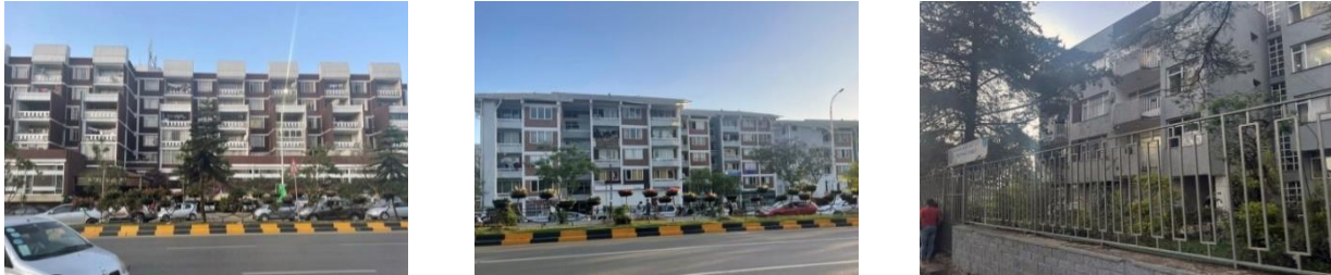
Figure 32: Presence of old buildings along Africa Avenue sidewalk
