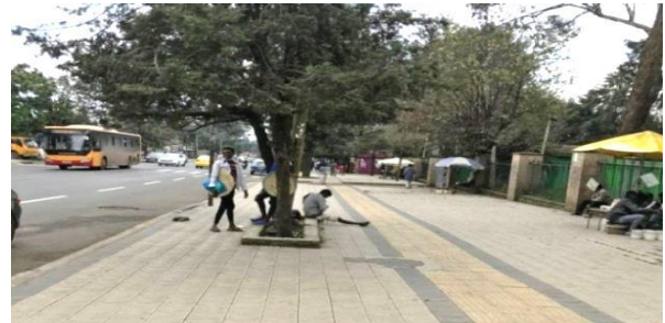
Figure 3: Pictures showing sidewalk of King George VI Street
