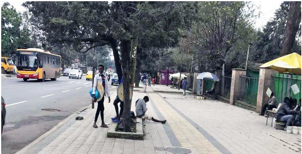
Figure 16: Pictures showing one of the segments of the King Gorge VI Street sidewalk
