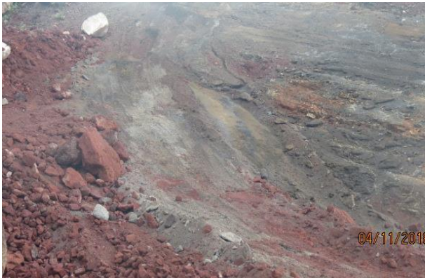
Red ash extraction site
