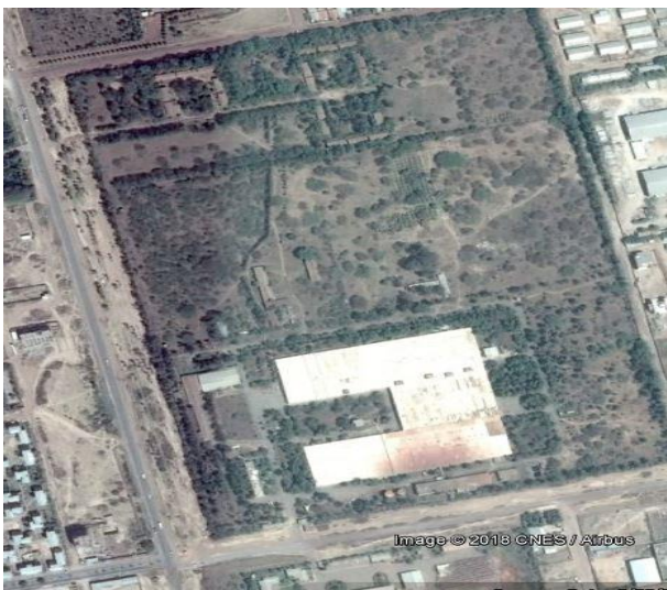
Large roof size (Hawassa Textile Factory)
