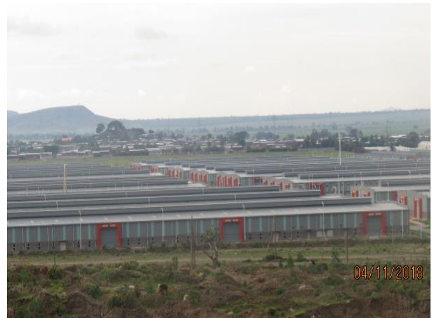
Hawassa Industrial Park
