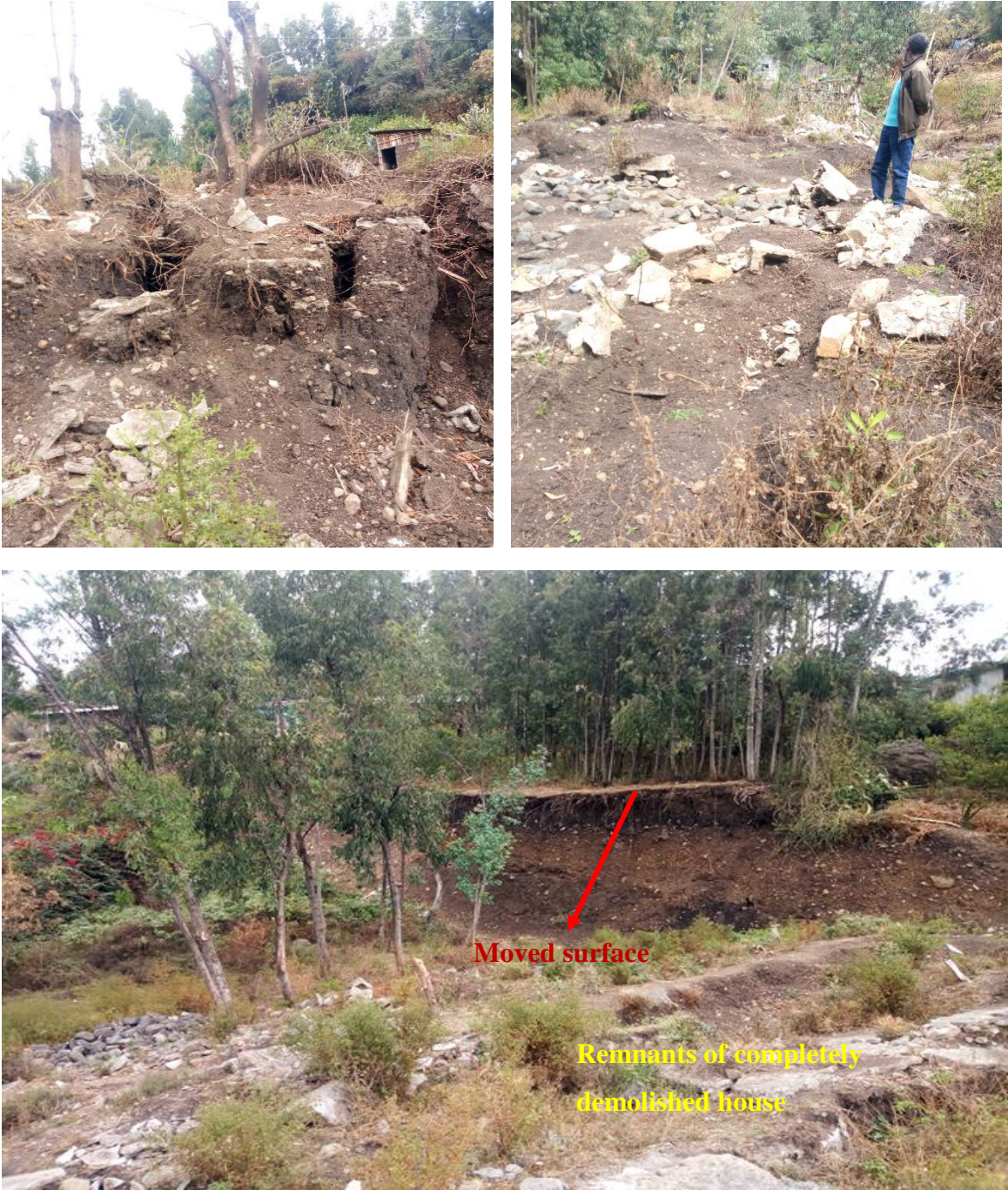
Figure 3.15: Demolished houses in Graar Genda
