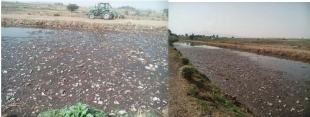
Figure 2: Kotebe wastewater treatment showing the mix of liquid and solid waste
