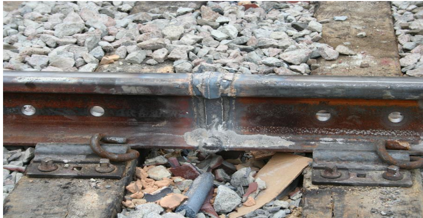
Figure 1.8: exothermic welding joint [11]
