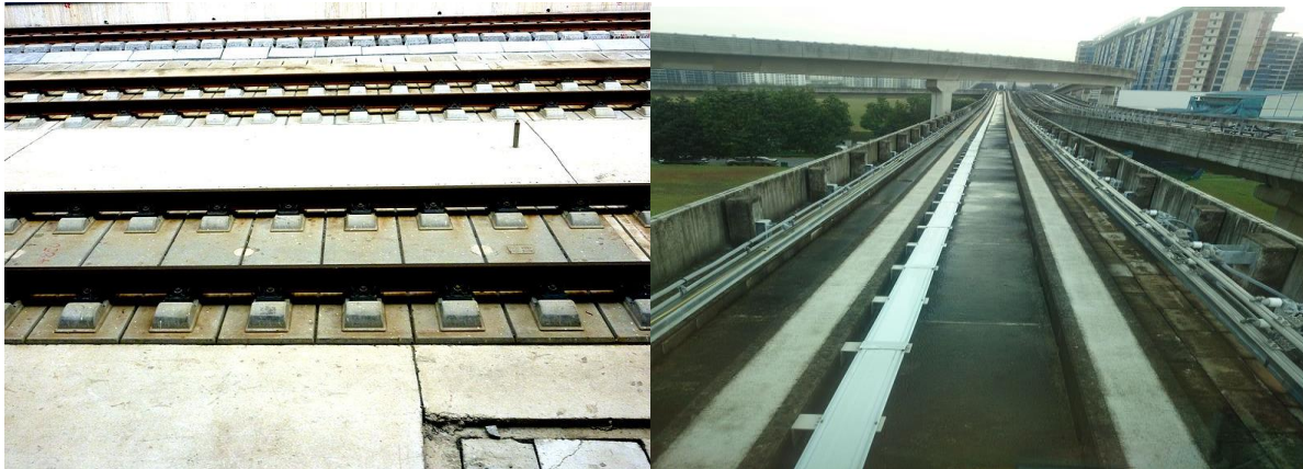
Figure 1.2: ballast less track [3]
