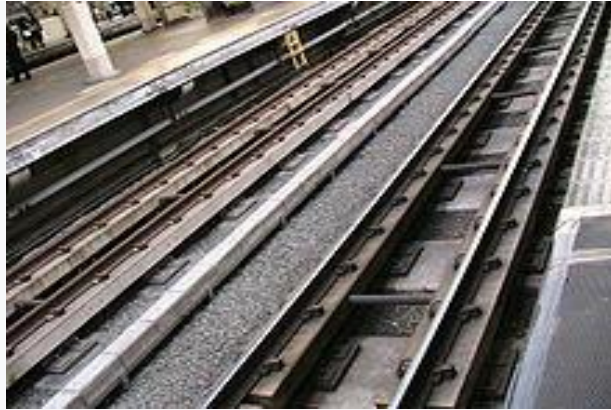
Figure 1.3: Ladder track at Shinagawa Station [4]
