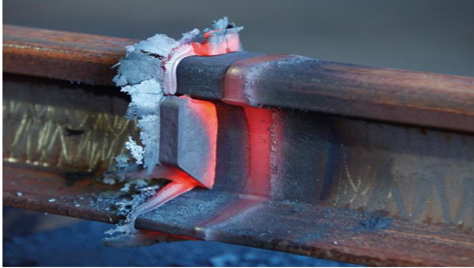
Figure 1.9: flash butt welding joint [12]
