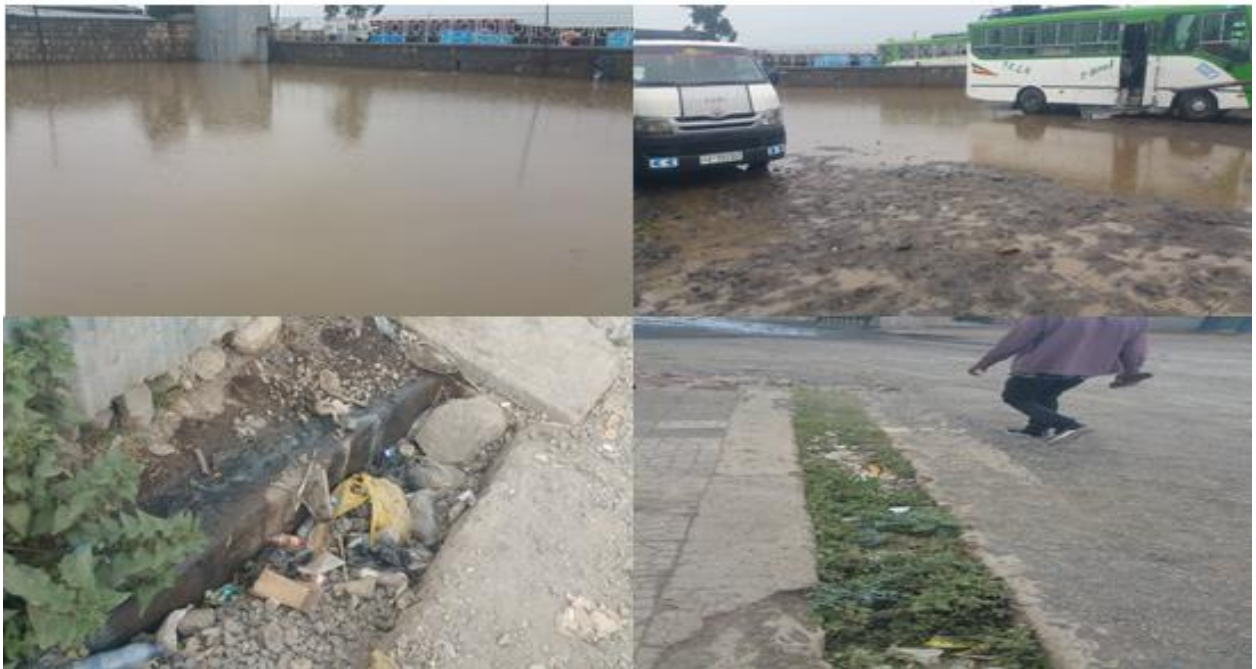
Figure 19: present drainage and flooding condition (site visit).
