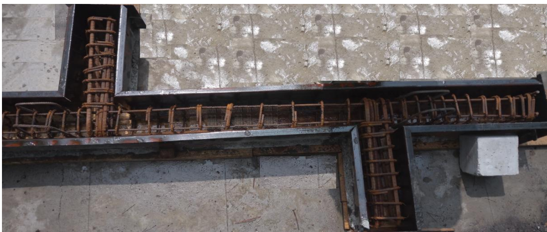
Figure 4-10 - Formwork with rebar (first stage)
