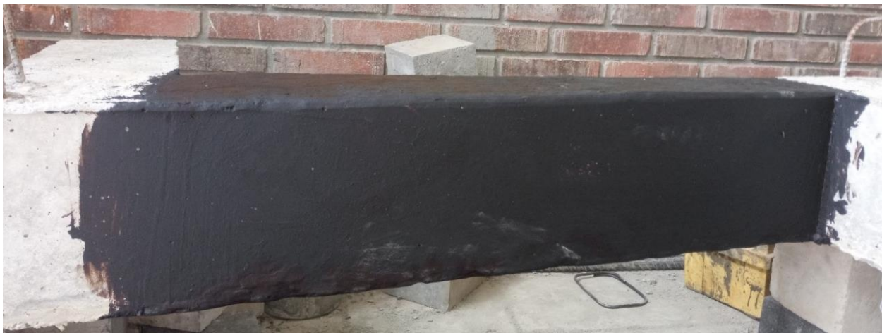
Figure 4-13-Primer on the substrate
