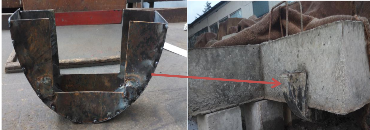
Figure 4-11 - Semicircular support formwork and second stage casting
