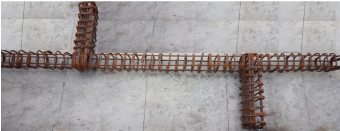
Figure 4-9 - Rebar cages (T50, 1)
