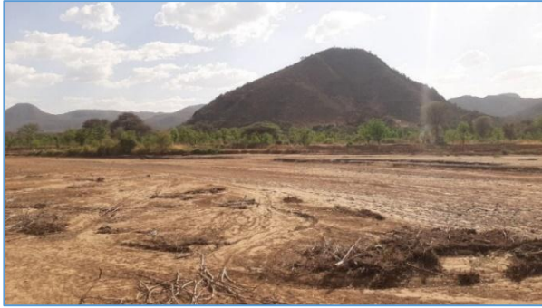
Photo 4 Right abutment of the dam
