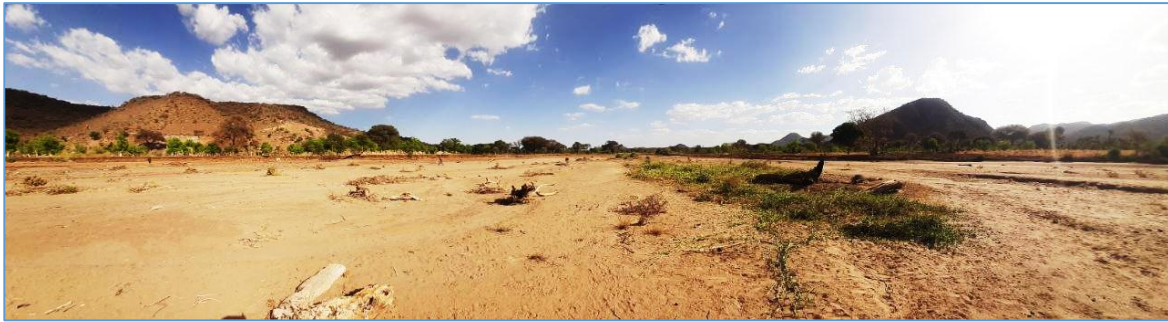
Photo 1 Upstream side view of the dam (Panorama photo from left to right Abutment)
