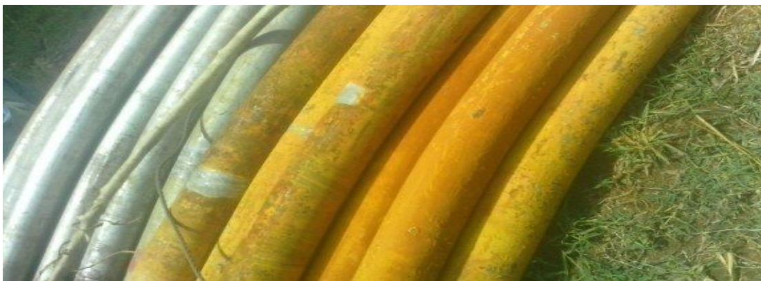
Figure17 The corroded pipe and the new pipe prepared for installing.
