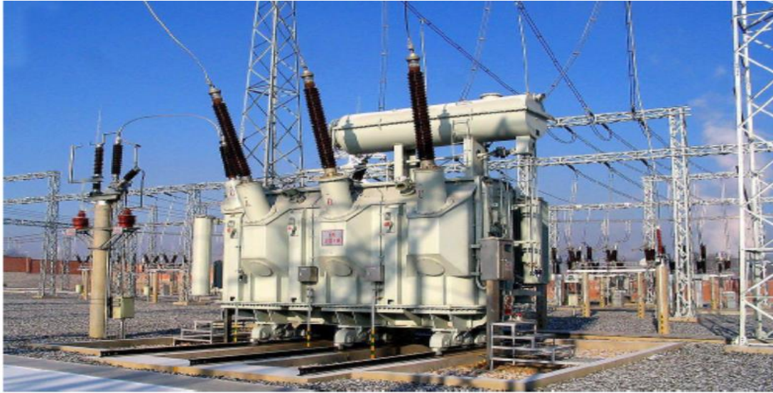
Figure 1: Typical three phase power transformer
