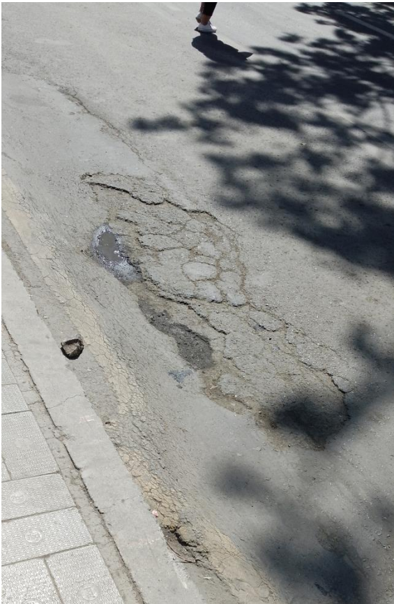
Figure 4.18: Potholes on the road, damaged road surface on the bus lane
