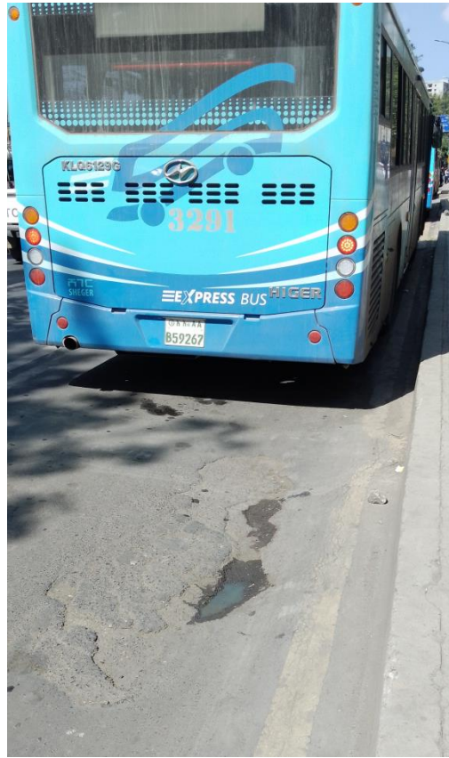
Figure 4.18: Potholes on the road, damaged road surface on the bus lane
