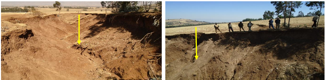
Figure 2.2: Gully erosion of the study area (photo from field observation)
