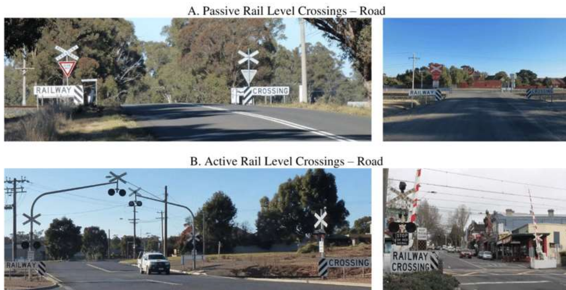
Figure 2-1: Level Crossing Control Type (Beanland, V., Lenné, M. G., Salmon, P. M., & Stanton, N. A. (in press) 2015)
