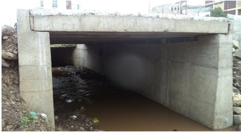
Figure 2.1-2 Railway Culvert at “Hayahulet”, Addis Ababa
