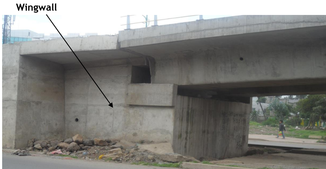
Figure 2.1-5 Railway Bridge concrete abutment
