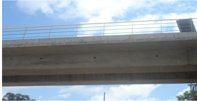
Figure 2.1-6 Double box girder concrete deck
