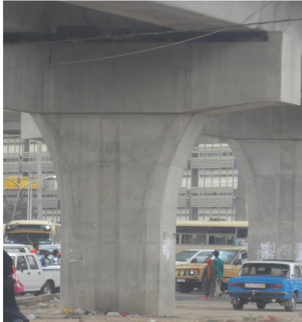
Figure 2.1-4 Pier column of railway bridge
