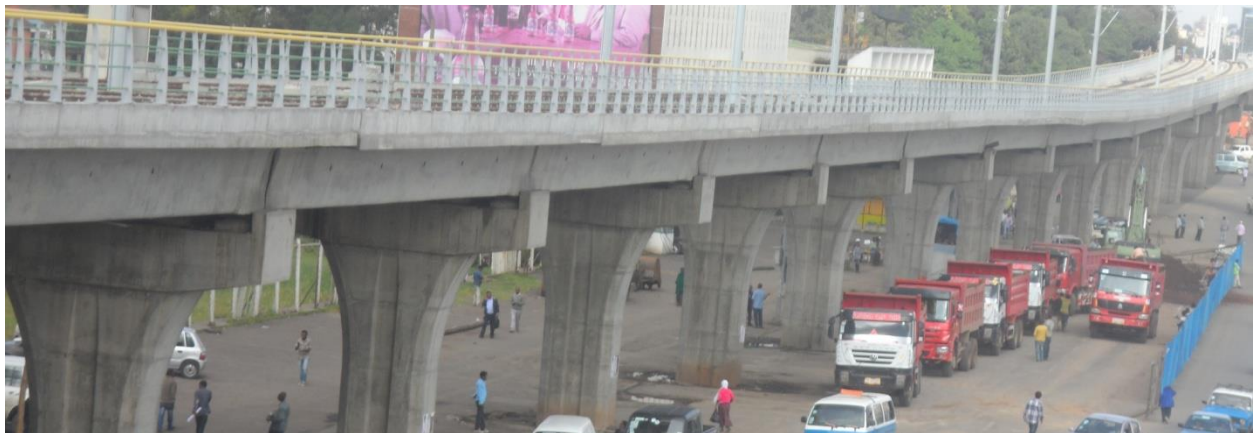
Figure 2.1-1 A Railway Bridge at “Meskel Square”, Addis Ababa
