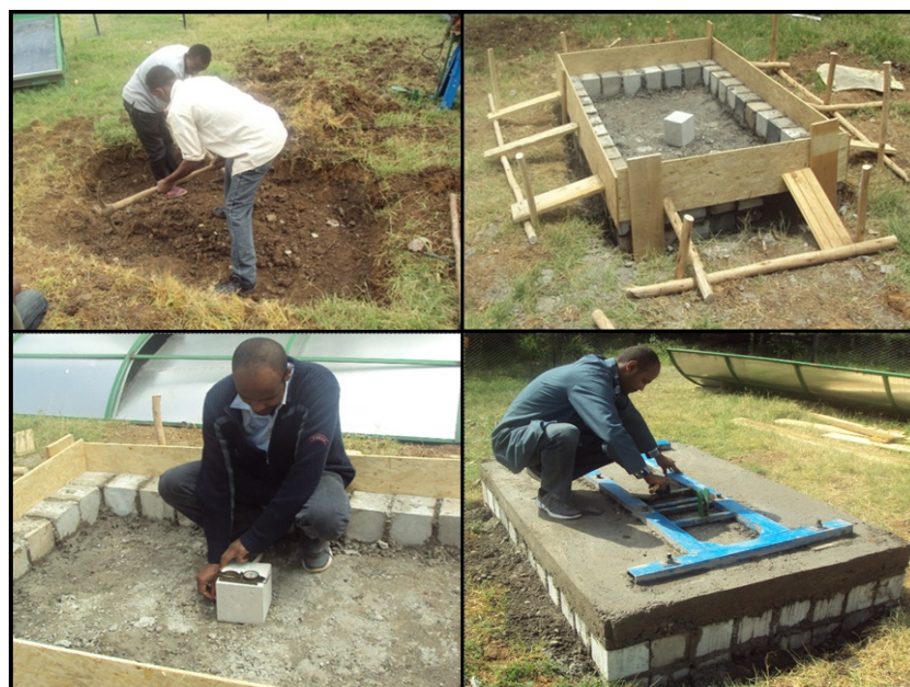
Figure 3.20 Foundation work of the parabolic trough
