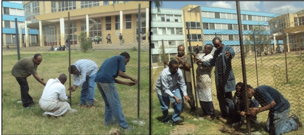
Figure 3.19 Fencing the selected site
