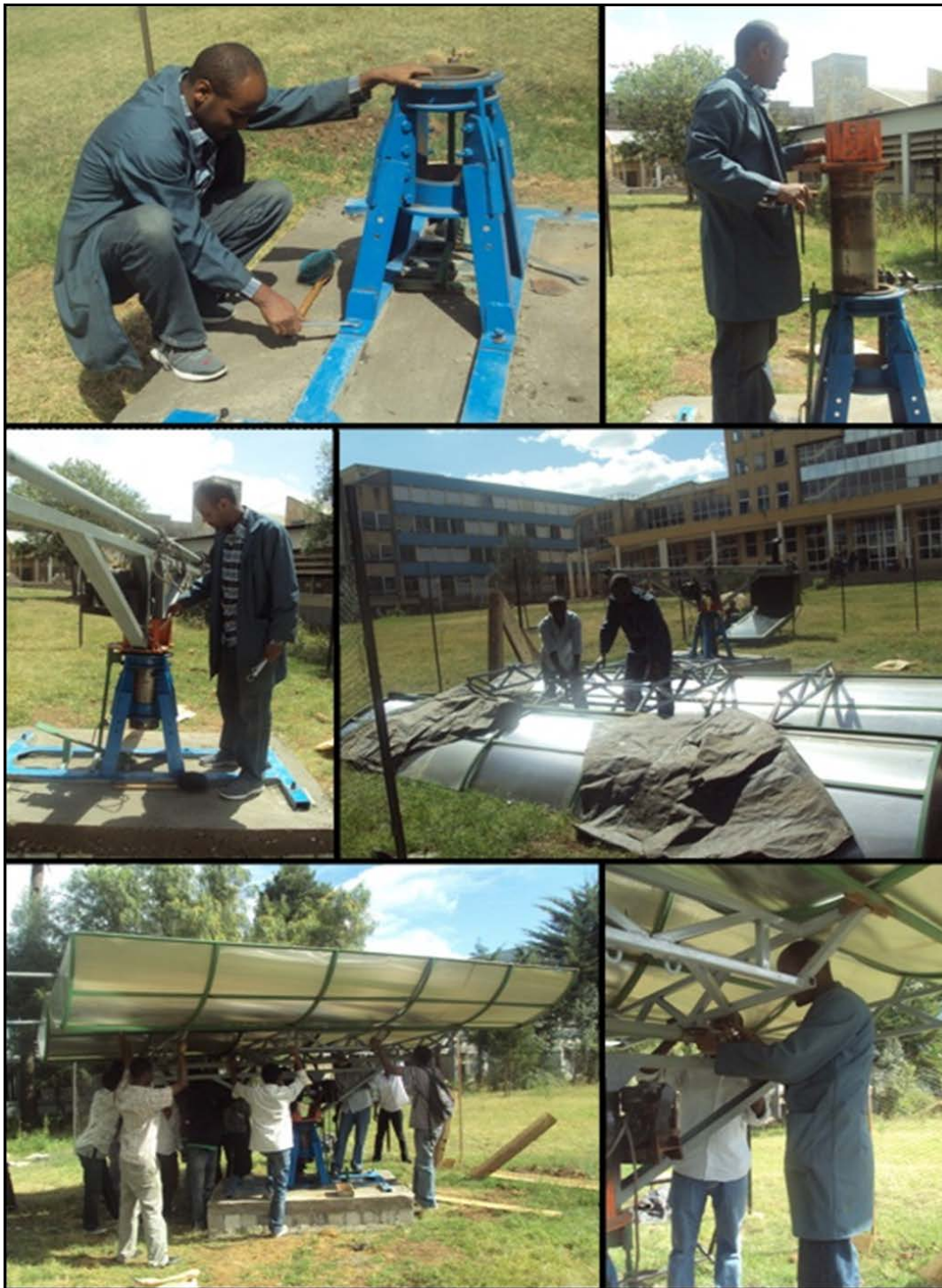
Figure 3.21 Installation of the parabolic trough
