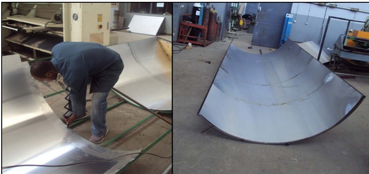
Figure 3.8 The parabolic trough structure covered with aluminum reflector
