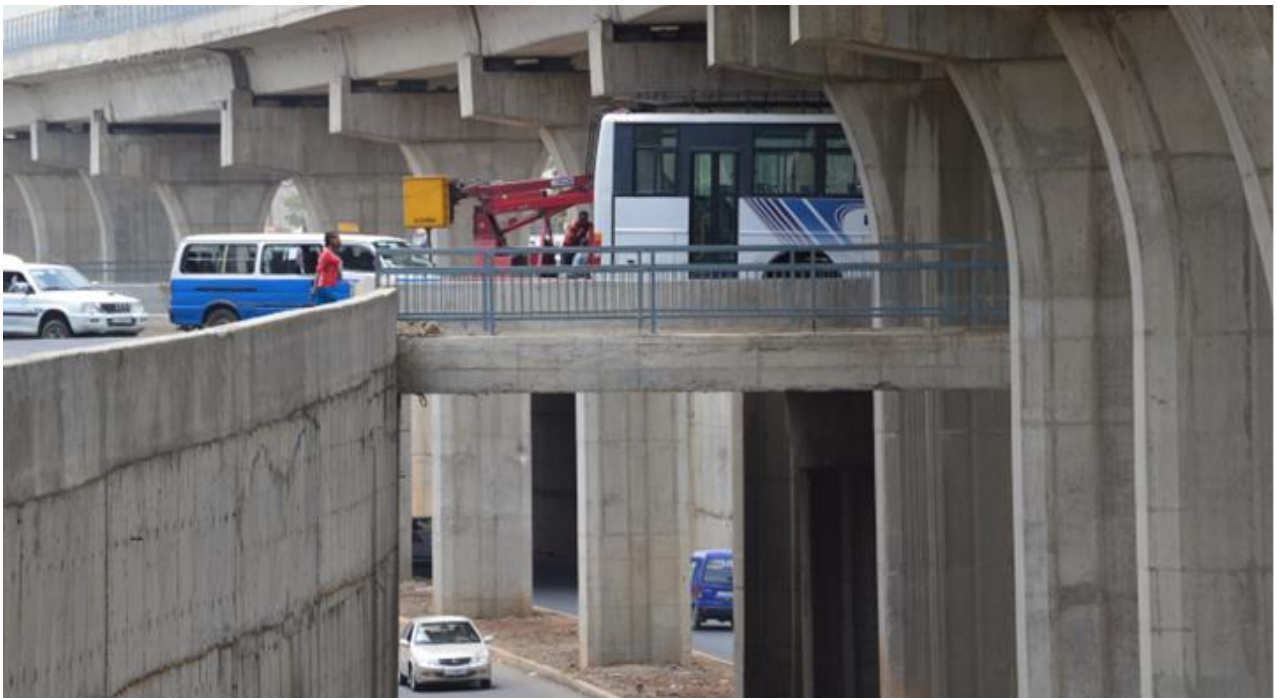
Figure -5.2: Addis Ababa Light Railway Transit Integration near Anwar Mosque Junction and near Mexico Square.
