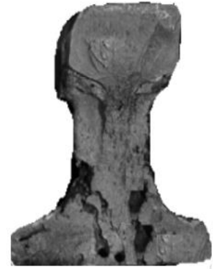
Figure 2.6: Fracture of a Thermic weld in the foot [17]
