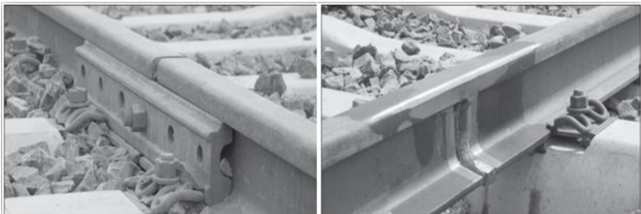
Figure 1.2: Rail joining with a screw (Left): Continuously Welded Rail (Right) [4].
