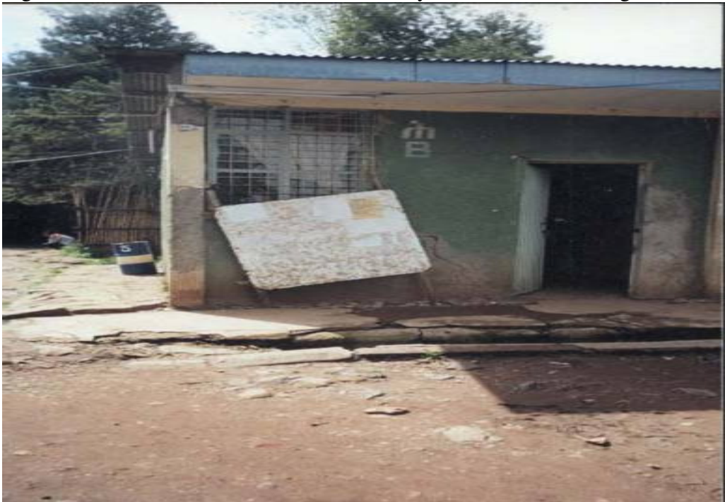
Fig 3.6 b Detachment of tie beam and column in bole senior secondary school
