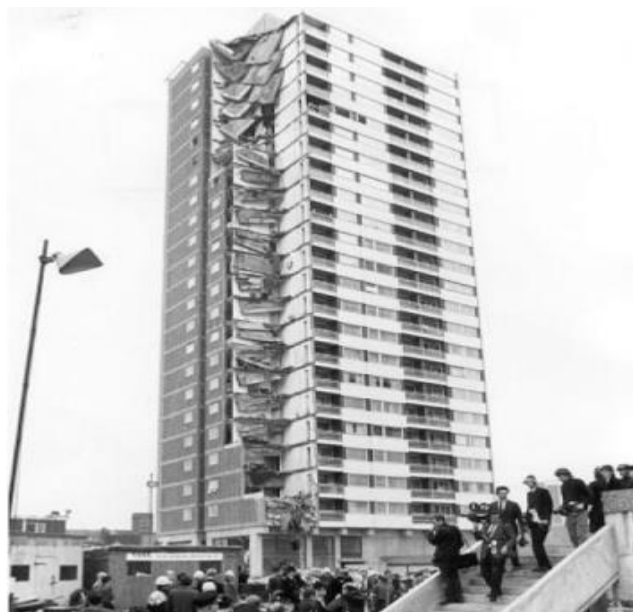
Figure 2.1: Ronan Point building after collapse (Pearson, 2005)
