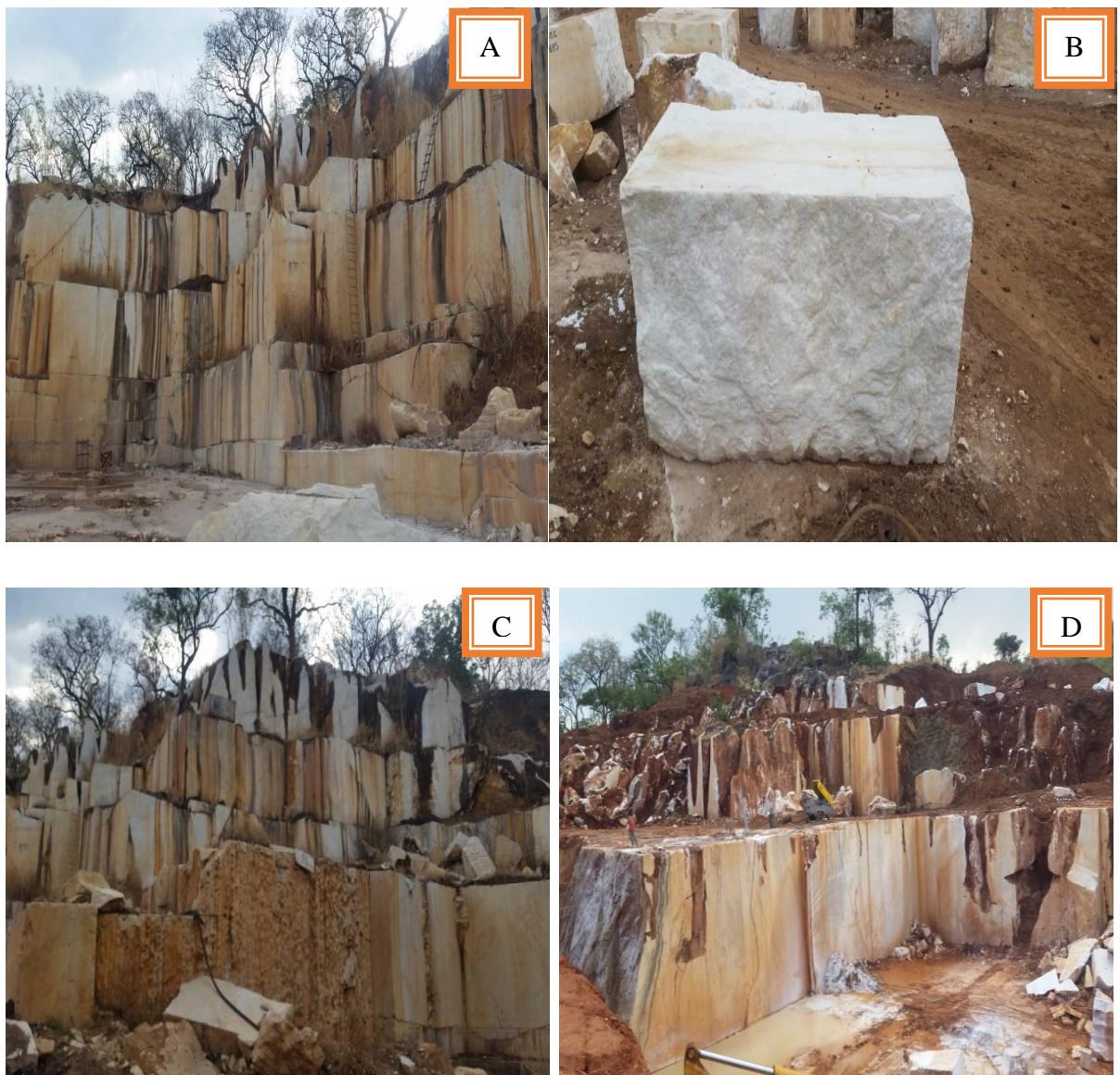
Figure 4.1: Daleti marble quarry site exposure in the northern part of the area.
