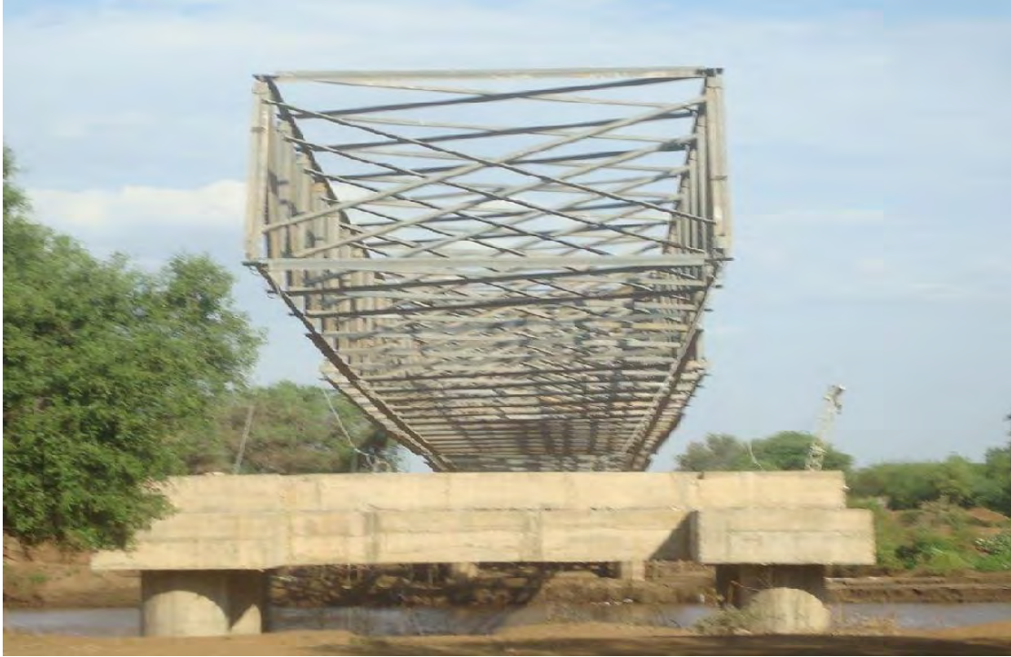
Figure 3.4: Tekeze River steel truss bridge
