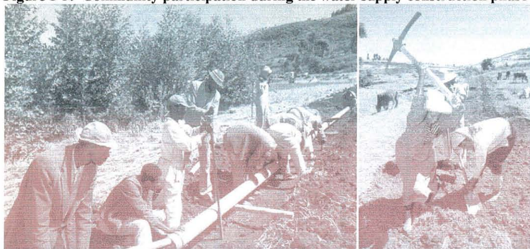
Figure 5-3: Community participation during the water supply construction phase
